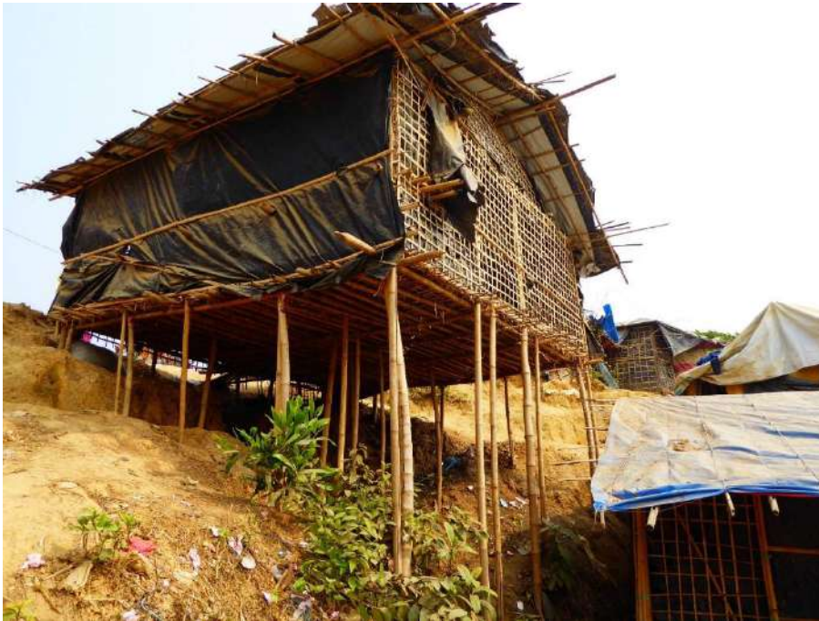
Left: shelter on stilts in camp, which is poorly constructed and has no vertical bracing. This is very vulnerable to wind, rot and flooding.
