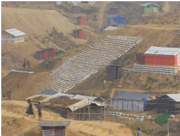
Above: Overly large, shallow wall
