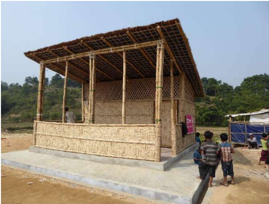
Left: bamboo walls fully exposed to driving rain due to very small overhang
