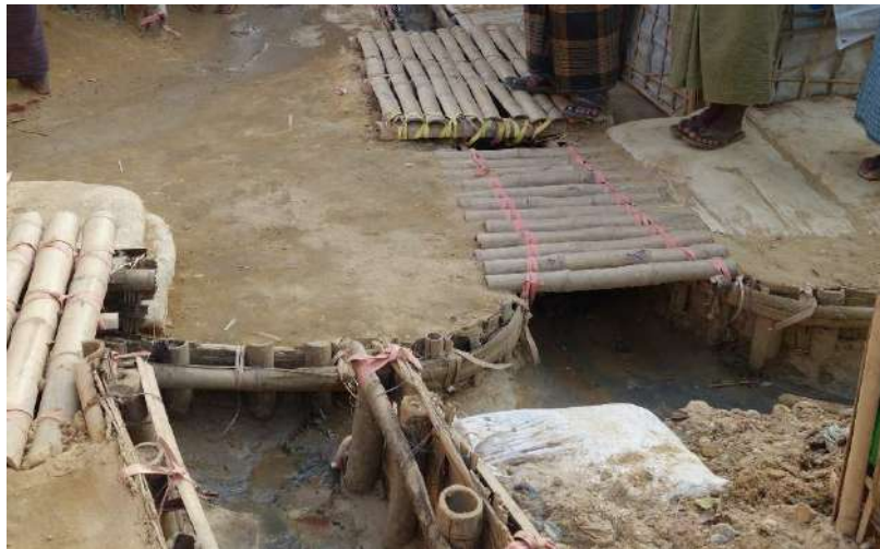
Above: Sudden changes in channel direction susceptible to erosion
