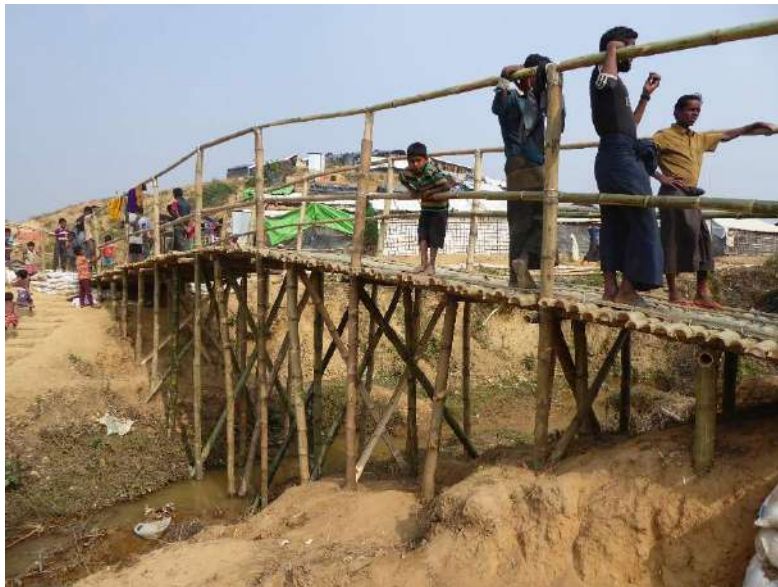
Left: placing bamboo directly into the ground, even if painted in tar and/or cast into concrete, will only last 6-12 months.
