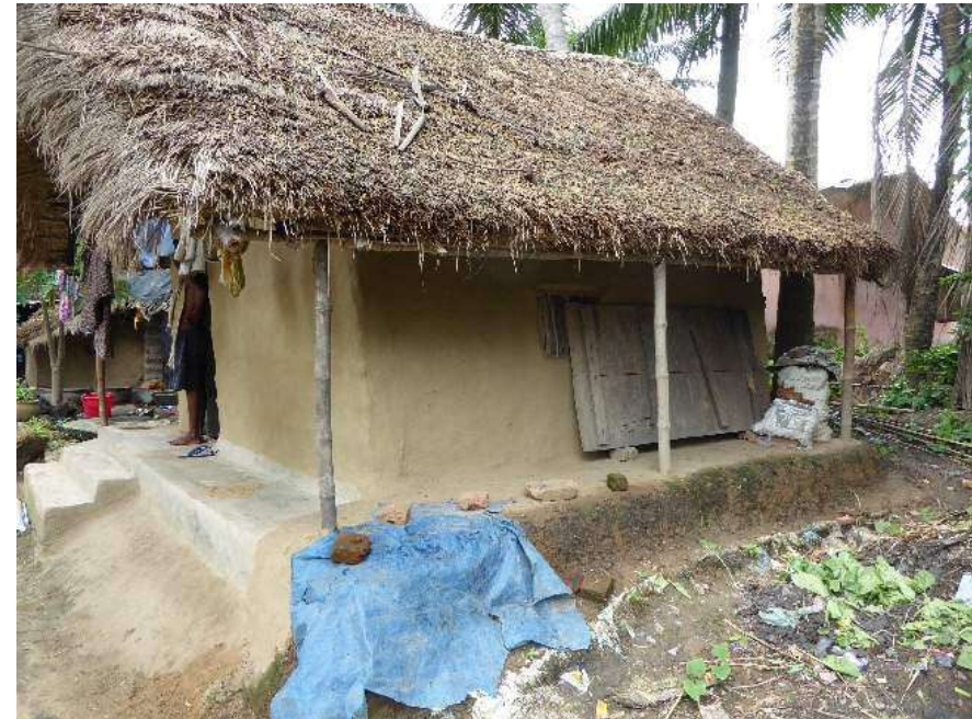
Left: bamboo walls fully exposed to driving rain due to very small overhang
