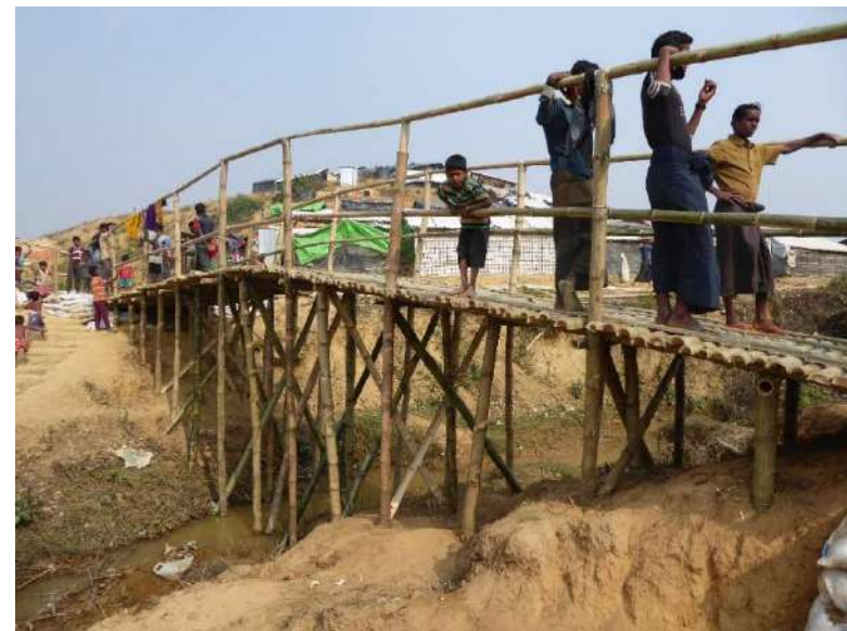
Bamboo bridge with closely spaced supports
