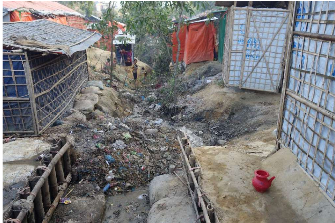
Debris collection along drainage channel
