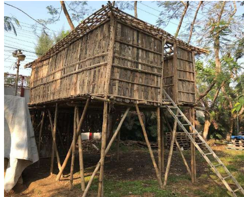
Left: shelter on stilts in camp, which is poorly constructed and has no vertical bracing. This is very vulnerable to wind, rot and flooding.
