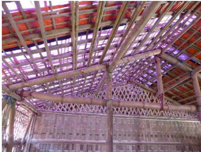
Above: borak as rafter has little benefit, double layer of muli has little benefit
