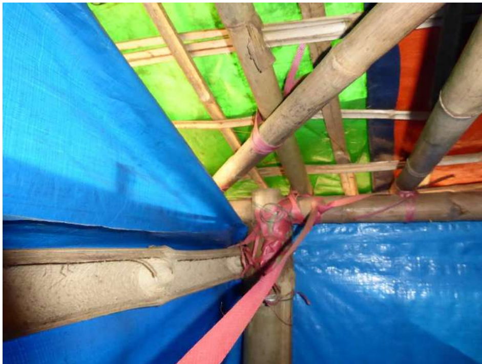
Above: small diameter or split bamboo being used for eaves is weak
