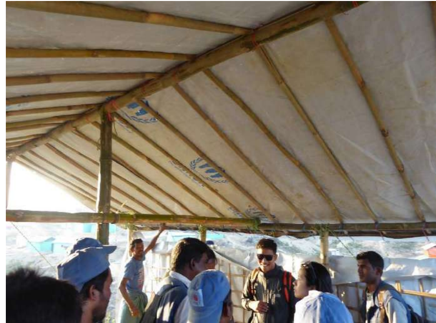
Above: borak as rafter has little benefit, double layer of muli has little benefit
