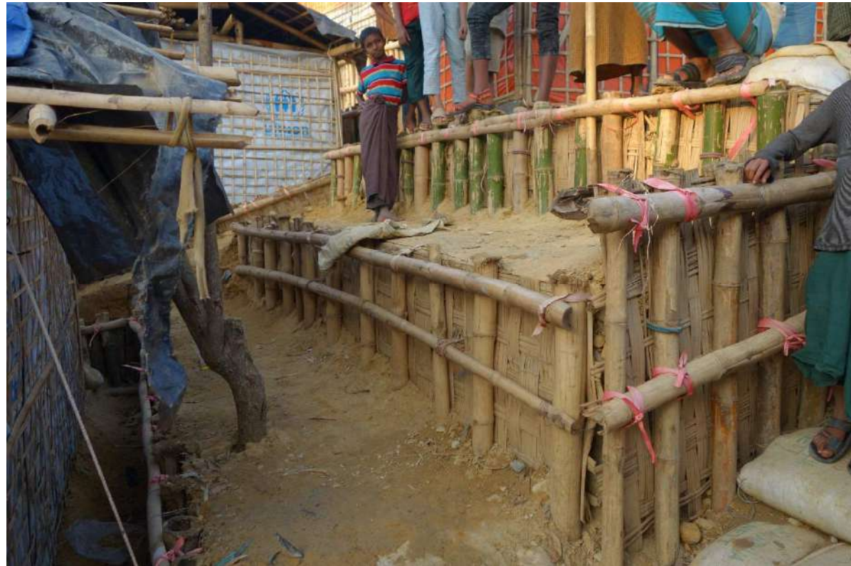
Stepped bamboo retaining wall
