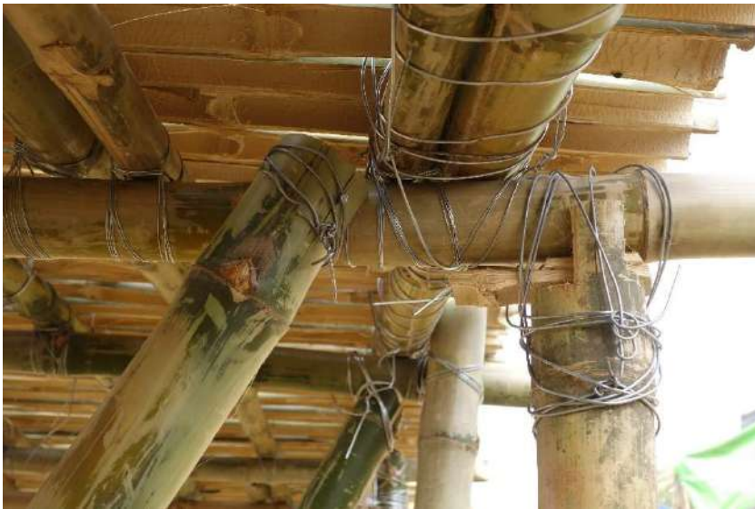
Top: existing bridge connection using metal wire which is weak and loose
