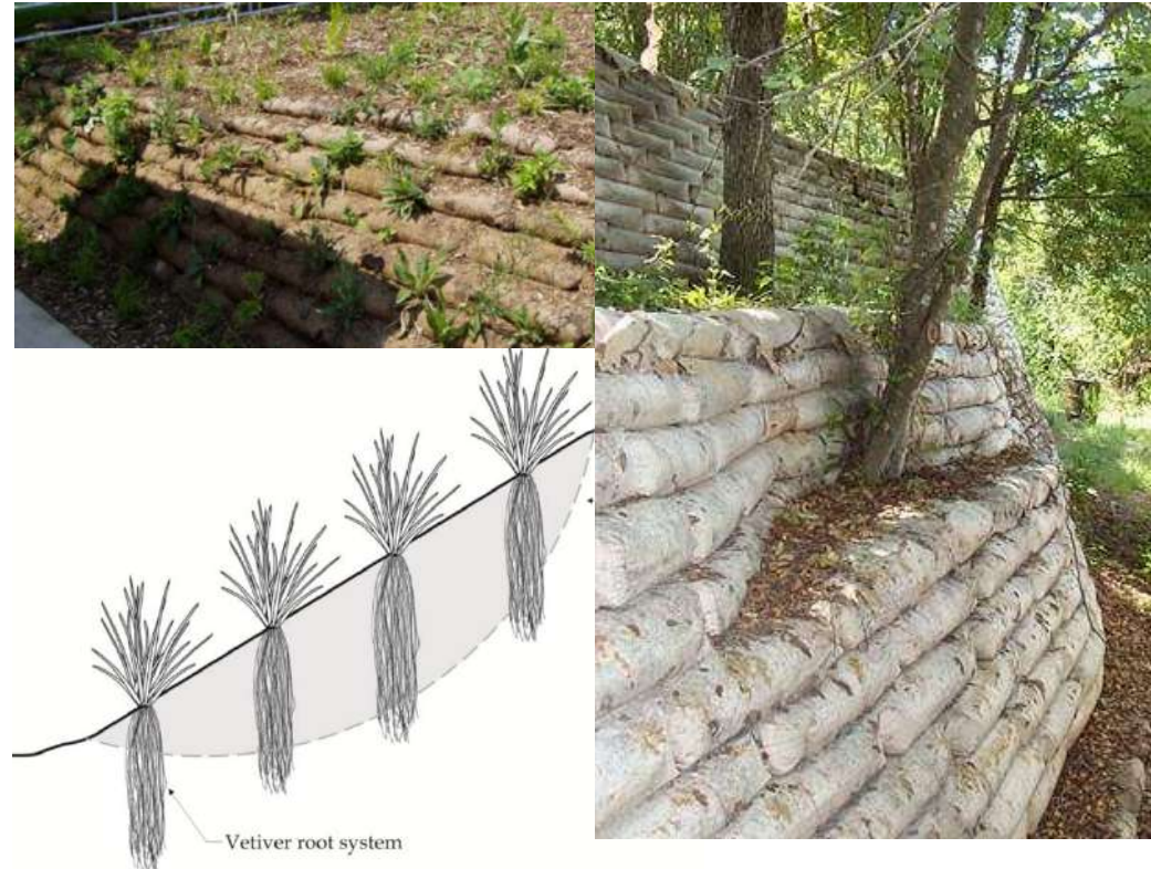
Above: consider seeded sand bags and replanting slopes
