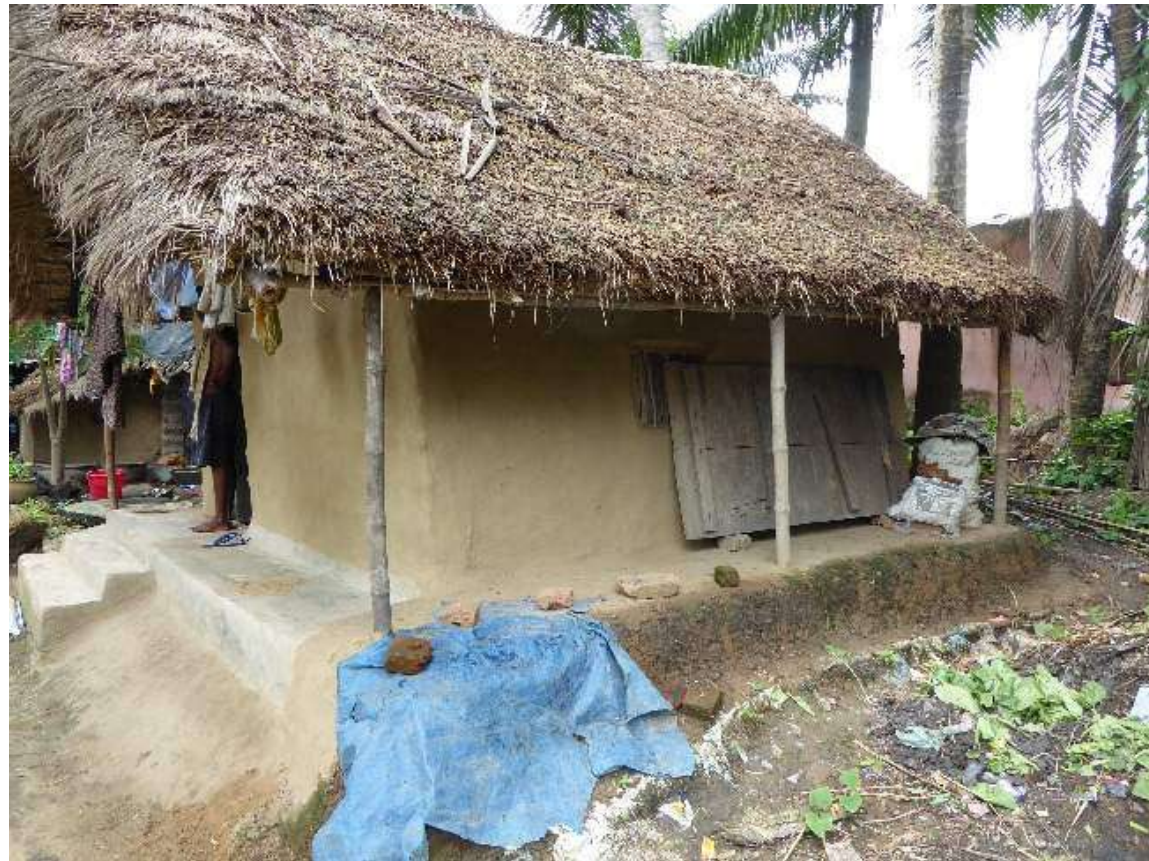
Traditional bamboo and mud house in India, with raised plinth to protect against flooding
