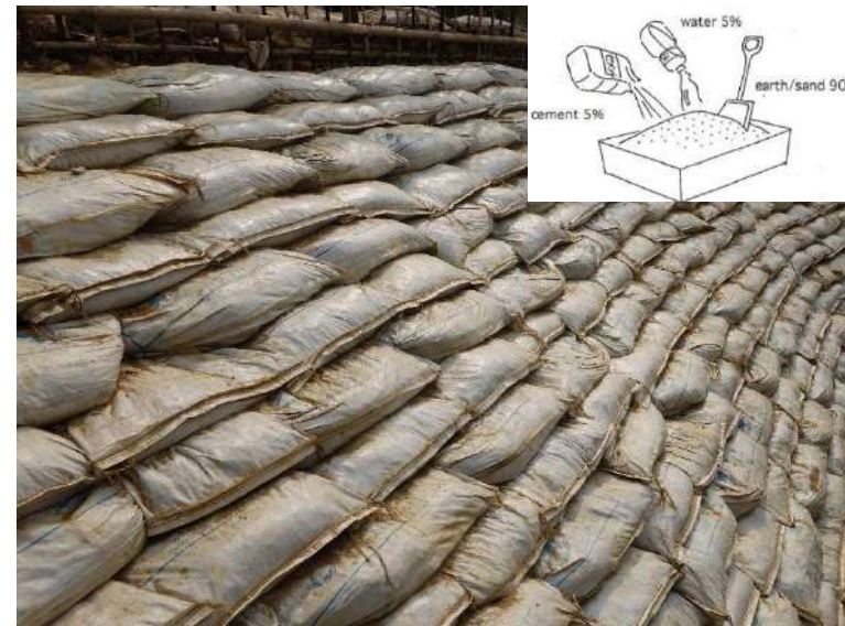
Above: consider better quality bags, stabilised fill material and planting
