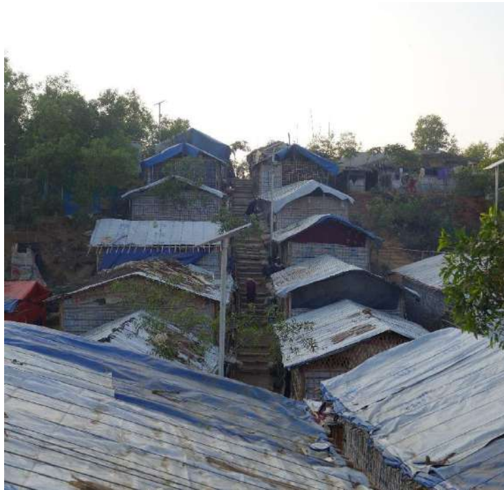
Above: Buildings should be orientated with long elevation inline with slope to minimise terrace height and extent.
