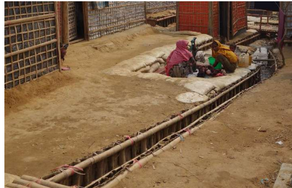
Above: Flush channel allowing easy water entry and ensuring better capacity due to greater below ground depth.
