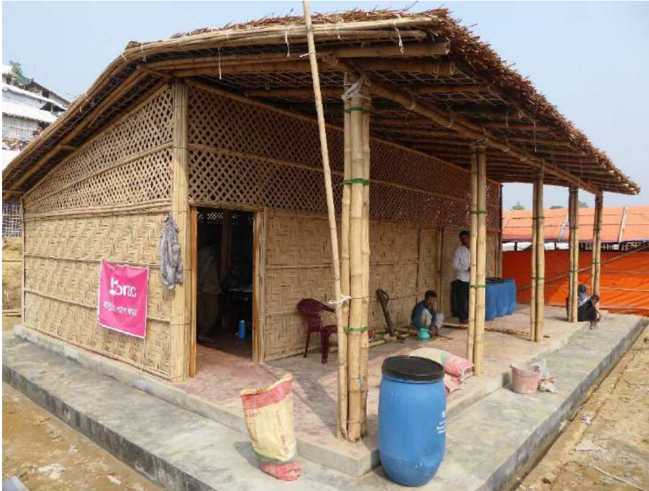
Left: external bamboo fully exposed to rain
