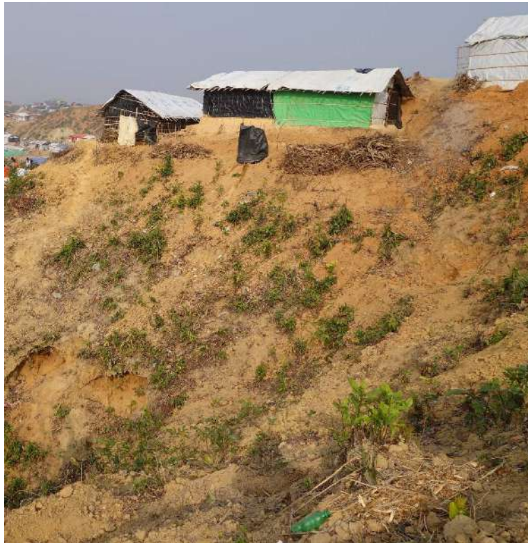
Above: Loss of natural slope stabilisation increases risk of landslides
