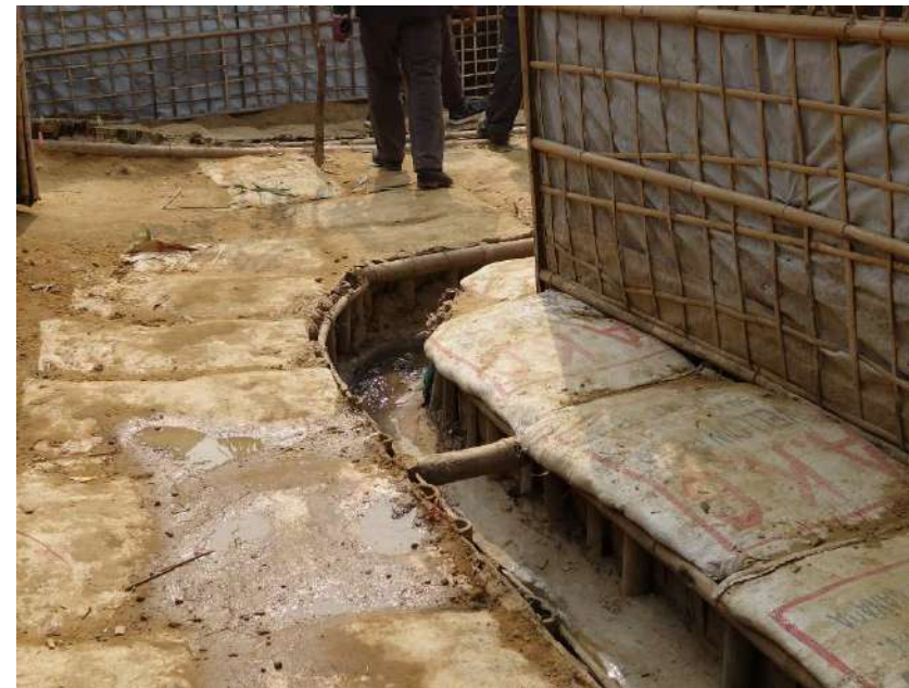
Above: Sudden changes in channel direction susceptible to erosion
