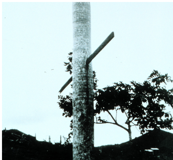
Figure 5: Hurricane wind damage in Puerto Rico 3
