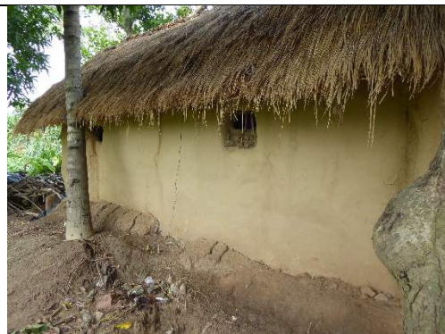
Figure 37: Veranda added to sides of house to protect against driving rain damage (India)
