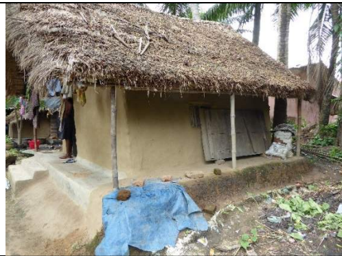
Figure 37: Veranda added to sides of house to protect against driving rain damage (India)
