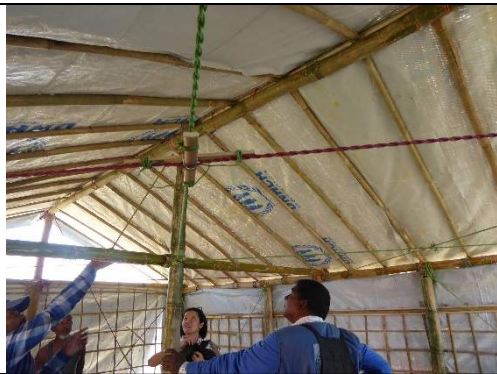
Figure 36: Allow the bamboo to breathe inside the waterproof envelope (Cox's Bazar)
