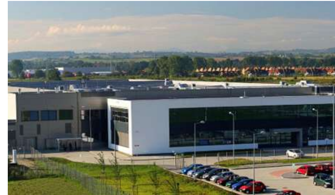
Somfy Electric Motors Factory, Niepołomice, Poland © Arup
