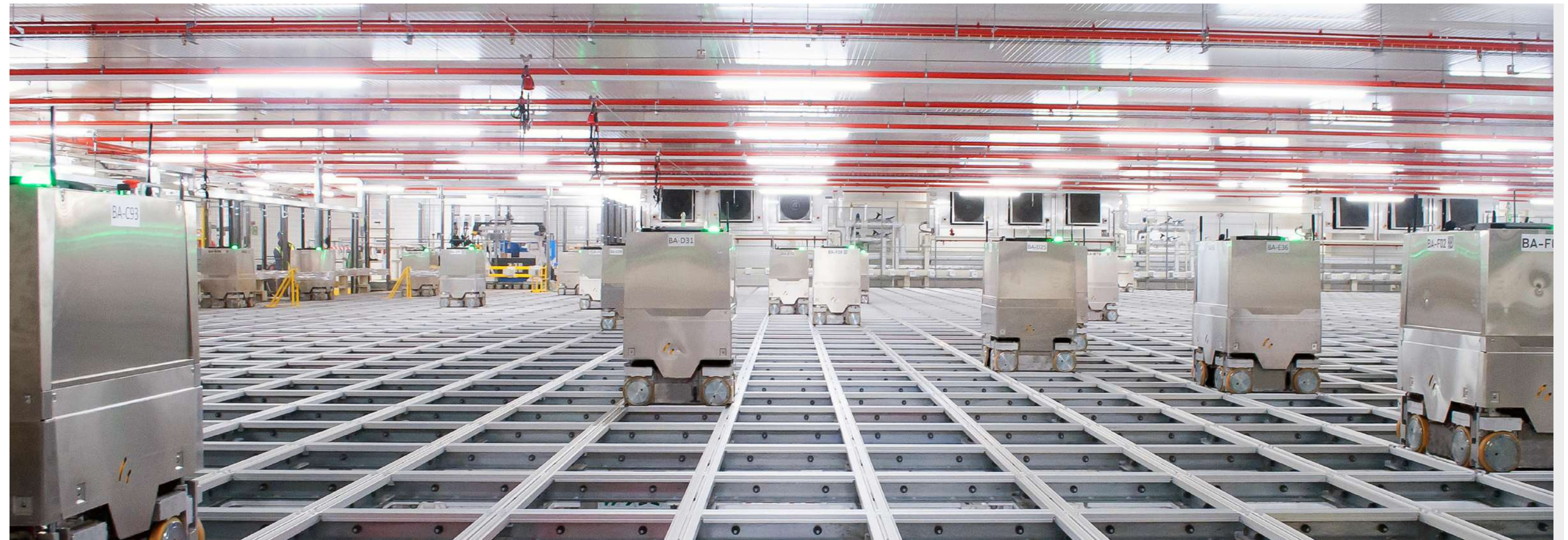
Ocado Distribution Centres © Arup
