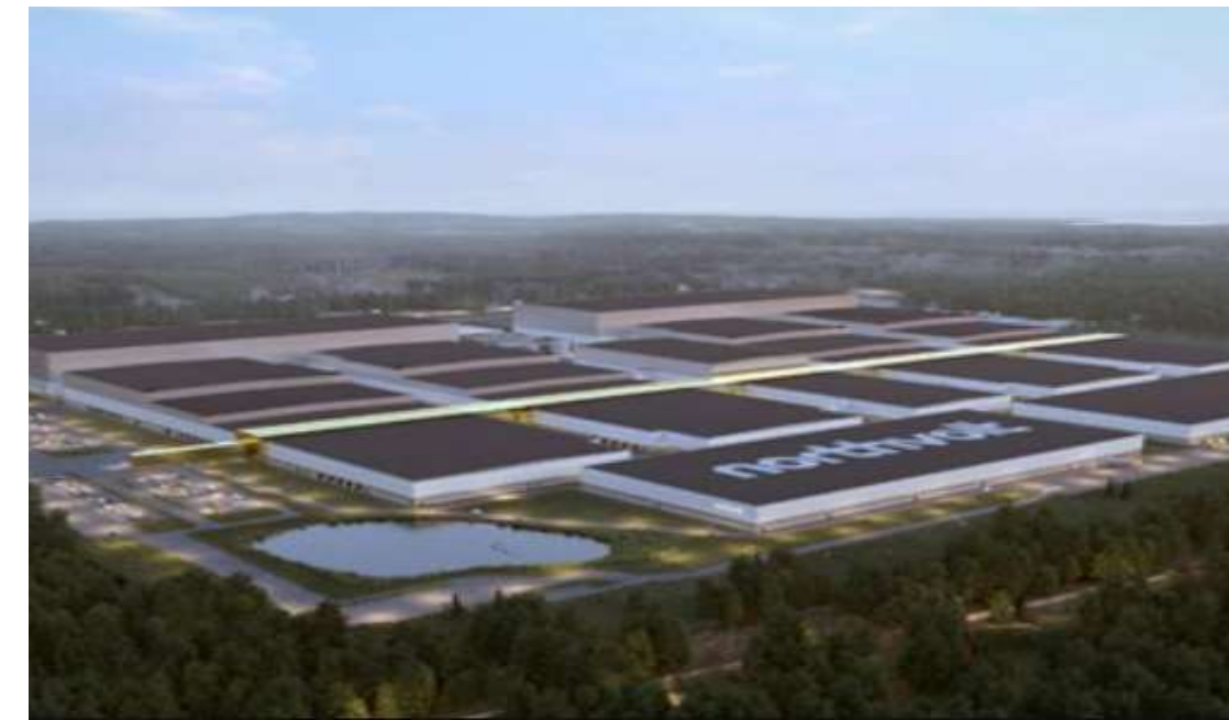
Northvolt Battery Manufacturing Plant, Sweden © Northvolt
