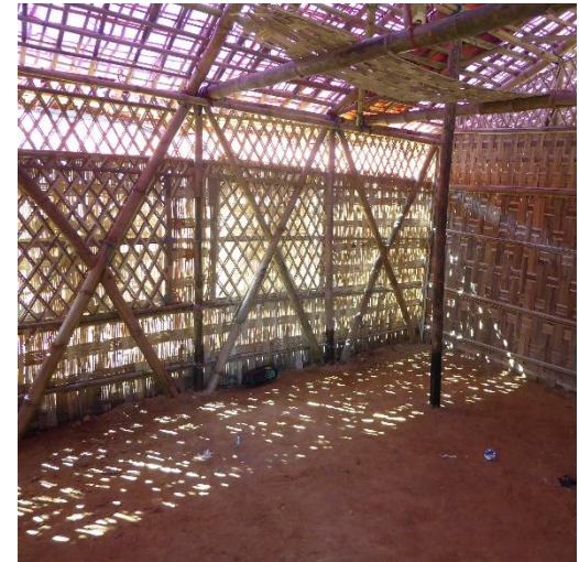
Smaller Existing Structures (Community Buildings or Halls)
