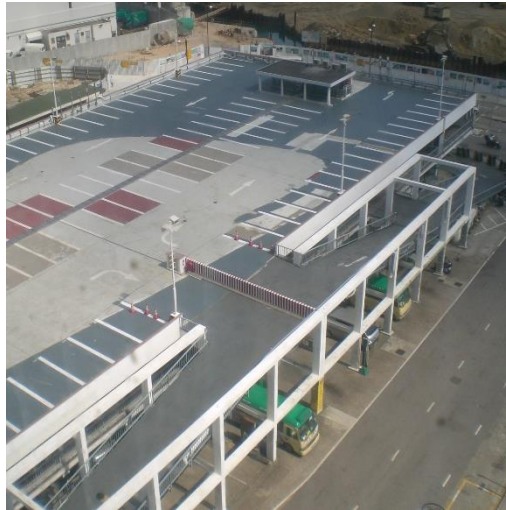
Confined Indoor Spaces (Multi-Storey Car Parks)
