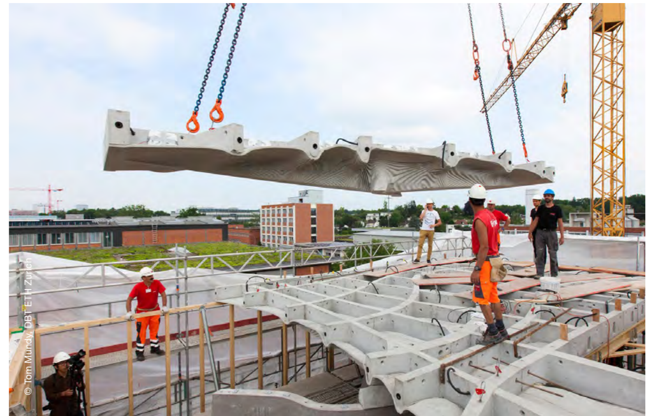
MATERIALS SAVINGS Installation of SmartSlab at DFAB HOUSE in Dübendorf, Switzerland. Manufacturing these slabs from 3D printed formwork (see page 27) enabled a staggering three quarters saving of material.
