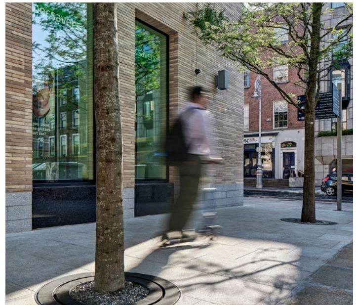
Renewal of granite paving on Molesworth Street, Dublin, by IPUT, to incorporate new tree planting, street widening and public bike parking.
