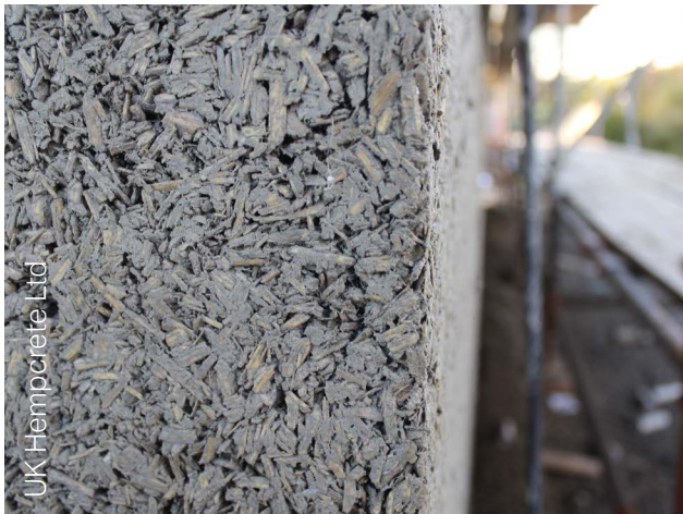
Figure 87: Example of hempcrete wall
