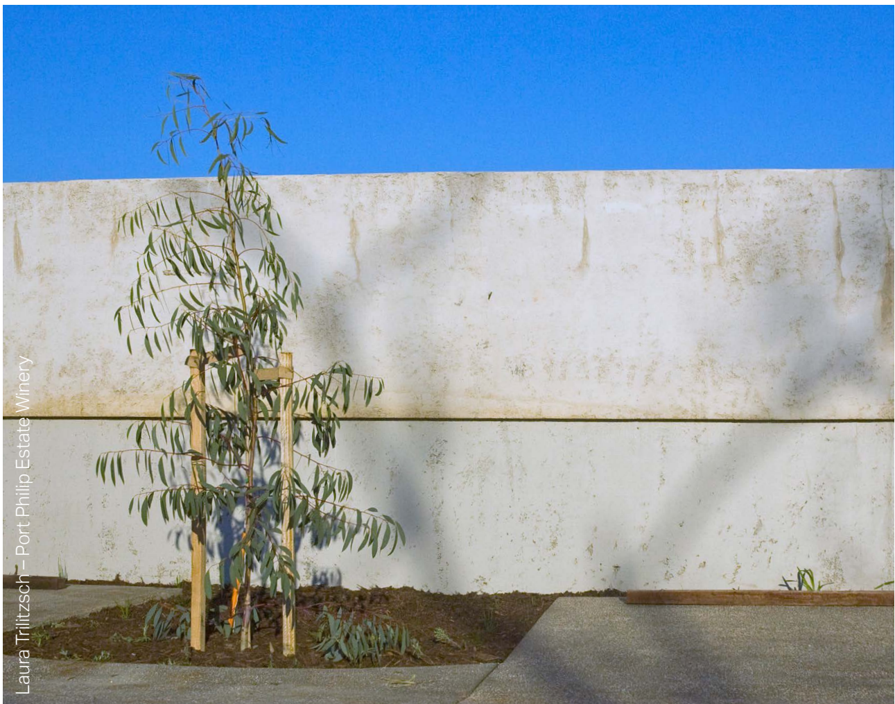
Figure 55: Example of rammed earth wall
