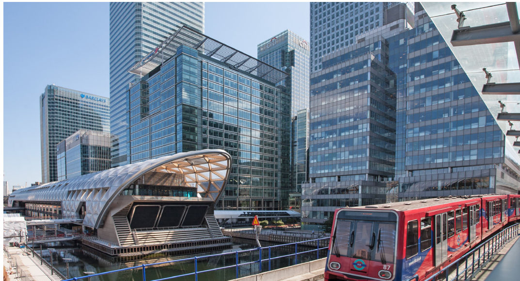
Canary Wharf Crossrail Station London, United Kingdom
