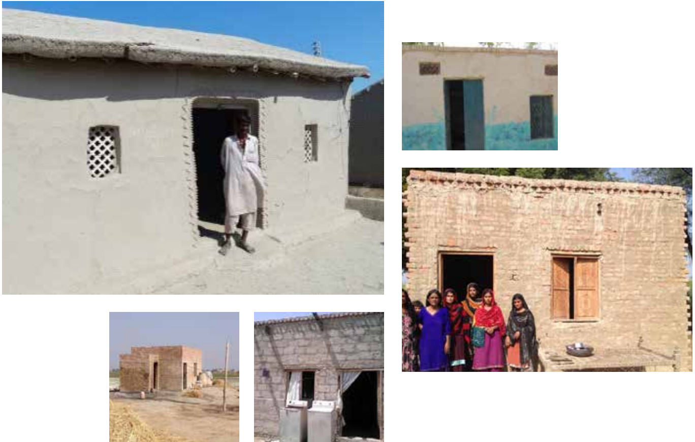
Figure 04. Shelter typologies (clockwise from top): loh kat, adobe, burnt brick, concrete block, burnt brick
