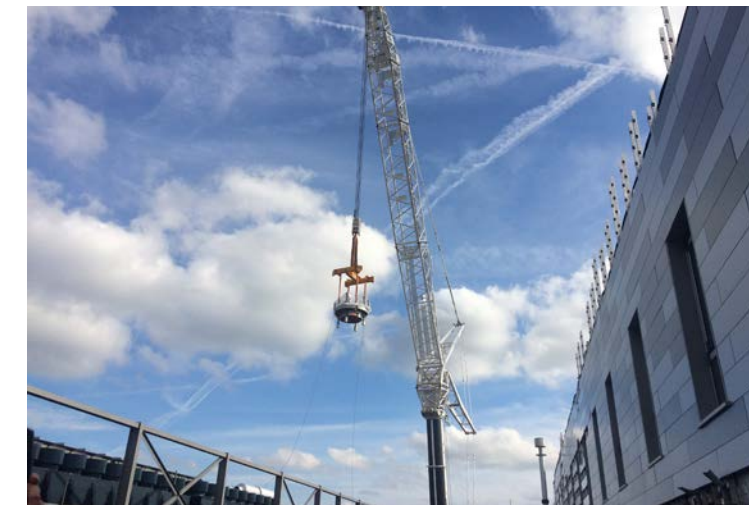
9: The cyclotron was lifted carefully into place using a large crane
