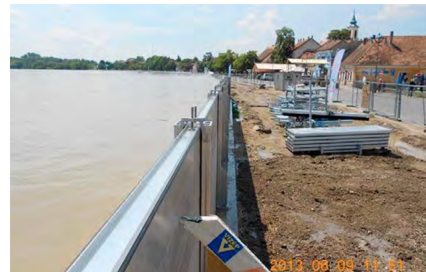
Establish a flood perimeter defense while limiting disruption to everyday operation by combining deployable barriers and permanent infrastructure.
