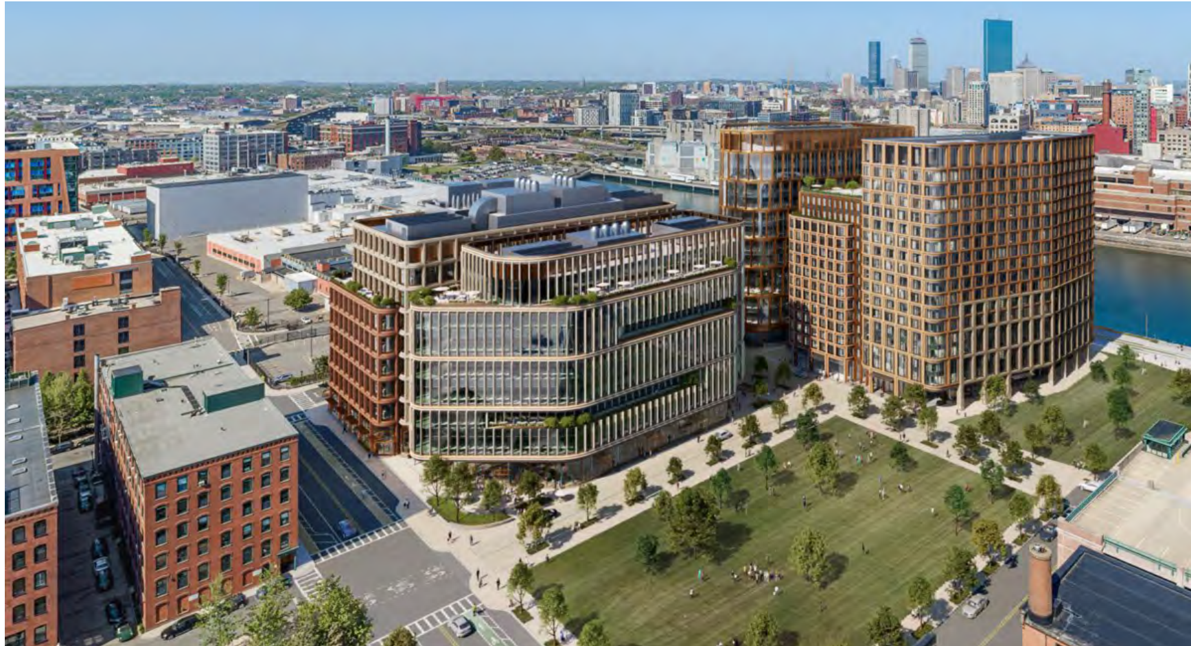
Arup provided structural engineering technical due diligence and site vibration assessment to determine the impacts to project feasibility of the traffic tunnel running under the site of Related Beal's proposed mixed-use development on the Gillette Channel-side site in Boston.
