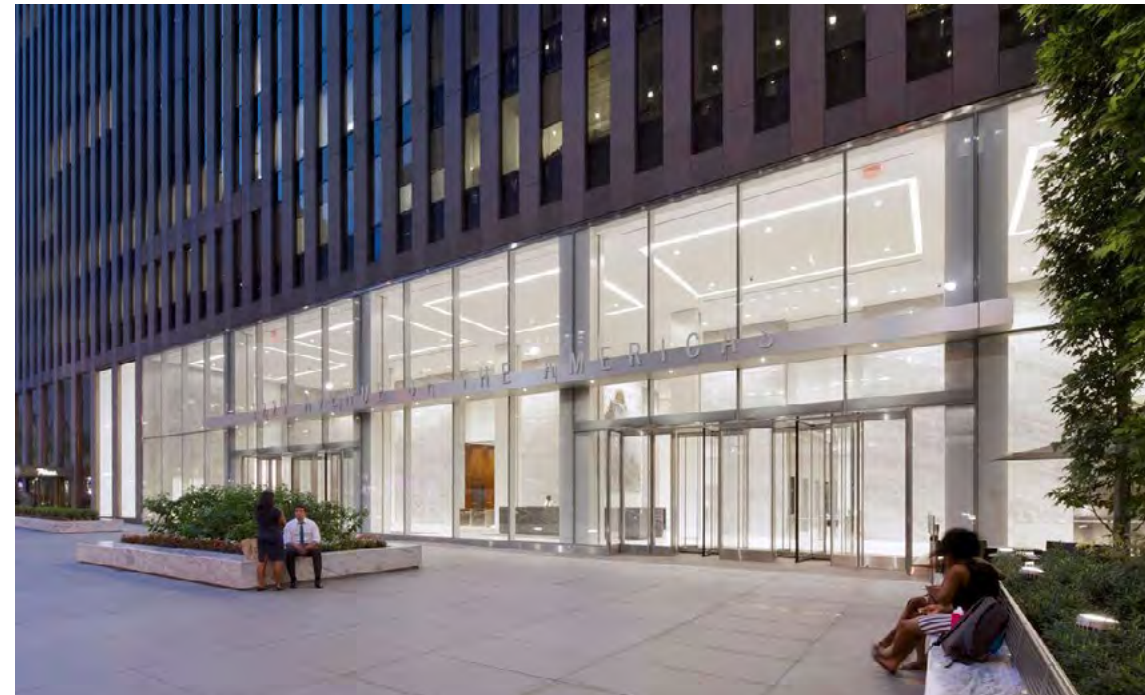
The repositioning of this historic tower’s lobby space created a transparent and welcoming entry for the tenants and emphasized the modernization of the building while providing comfort and maintaining the US Green Building Council LEED EB certification.
