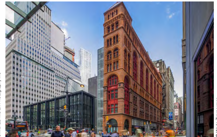
For the Corbin Building renovation in New York City, Arup developed repair techniques that allowed for most elements of the building to remain in place during the restoration of its exterior brickwork, stonework, and cast-iron façade. By retaining a watertight shell, restoration was completed ahead of schedule at a reduced cost.
