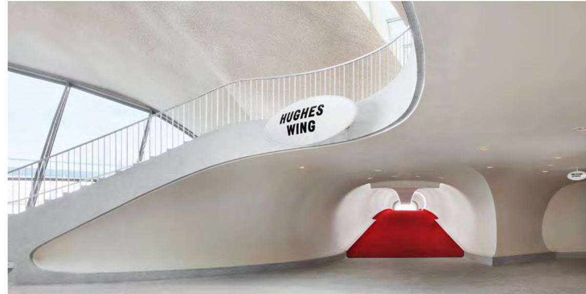
The existing TWA Flight Center had non-conforming stair treads and guard rails, extended travel distance and no sprinklers at the main roof.
