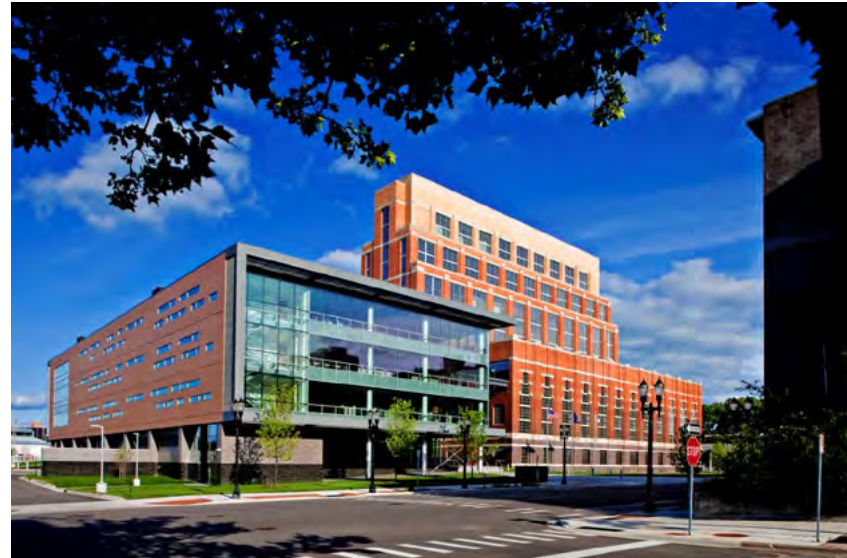
The award-winning conversion of a coal burning power plant into Class A office space was achieved by rationalizing the plant's existing floor plates, which doubled the lettable space while preserving the building's unique character.
