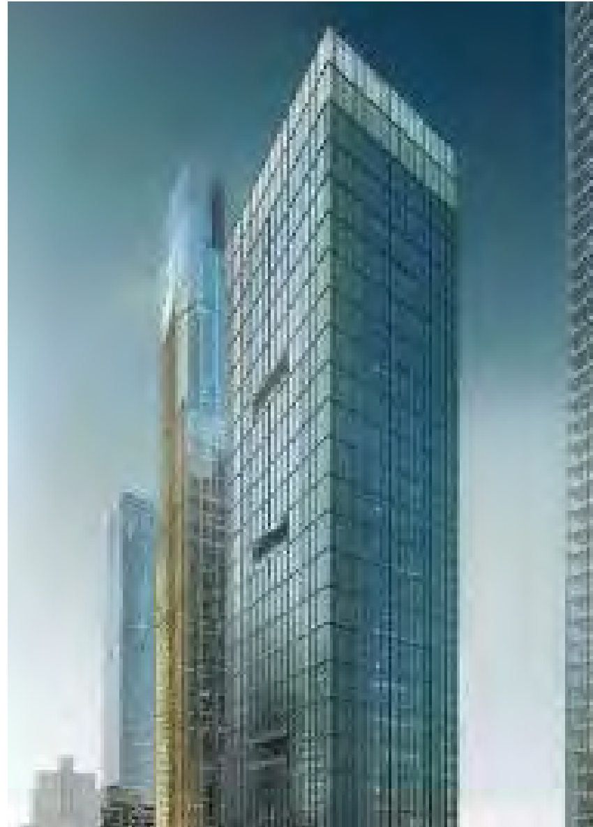
Arup provided structural engineering technical due diligence and value engineering review to support Mitsui's $1B investment in Related's 55 Hudson Yards project in New York City.
