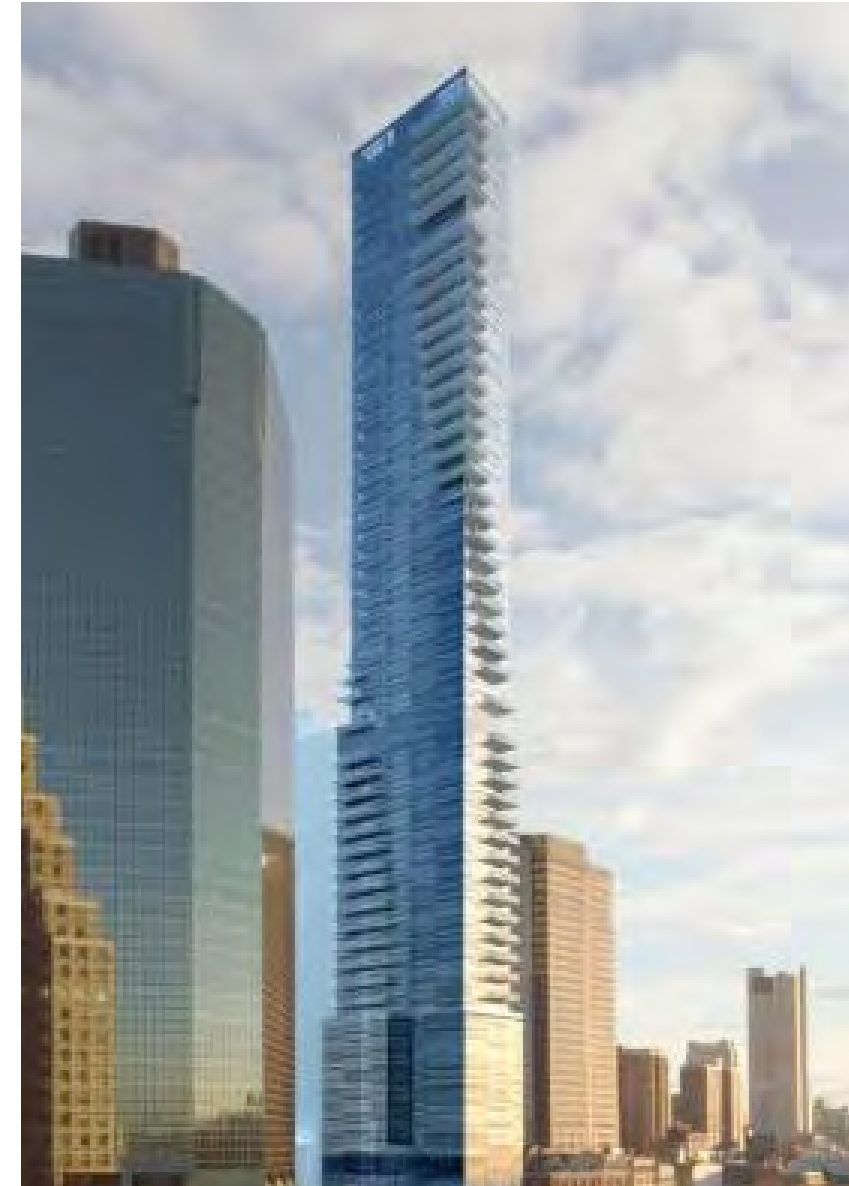
Arup provided structural, wind, and geotechnical engineering peer review and forensics analysis to assess Fortis Property Group's tower under construction at 161 Maiden Lane in New York City.
