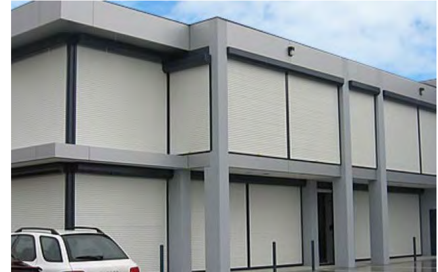
Retrofitting temporary or permanent hurricane shutters to prevent building envelope penetration in extreme winds.
