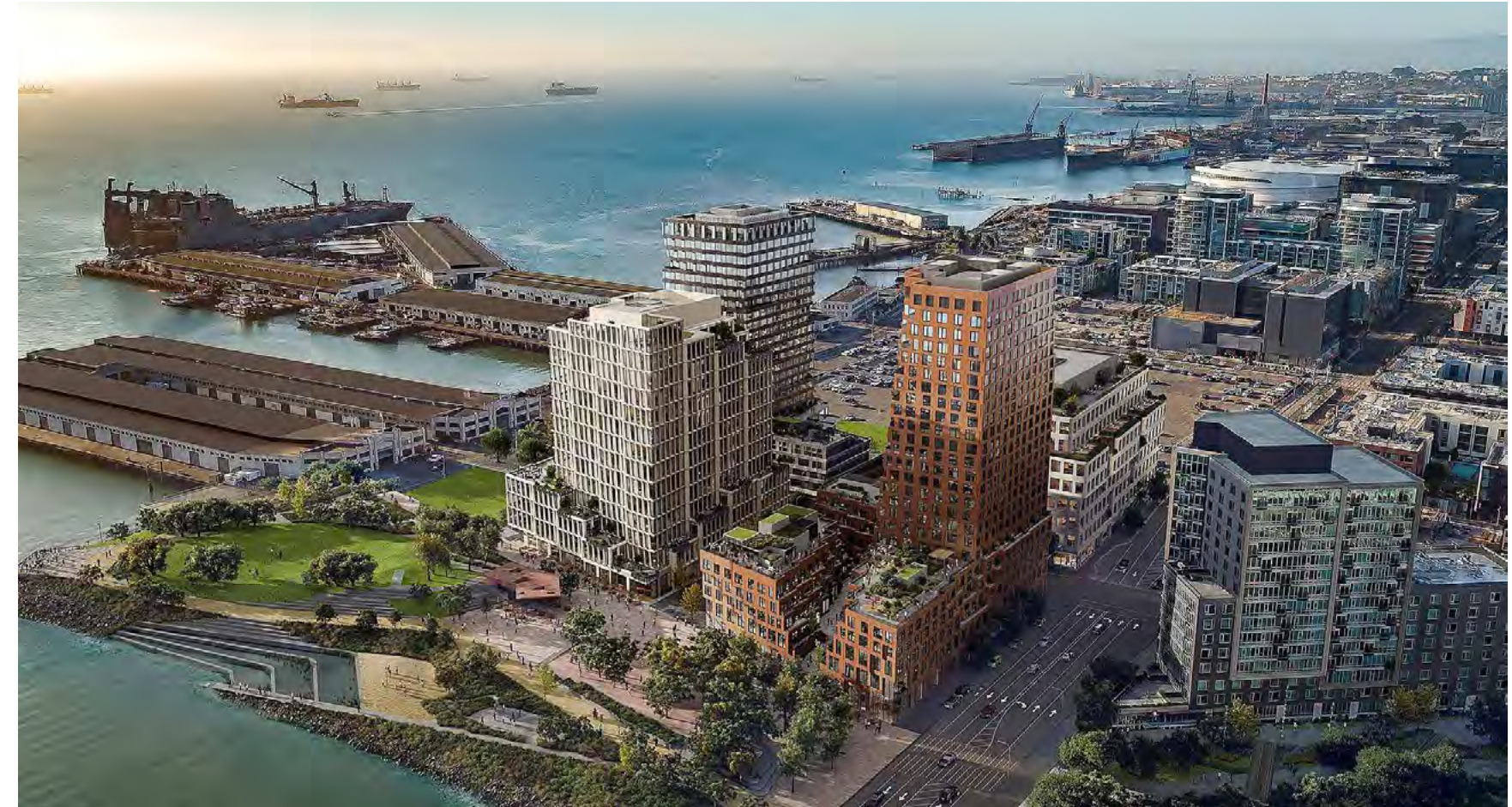
Arup provided structural, geotechnical, and seismic engineering technical due diligence and site assessment advise to help Mitsui Fudosan assess risks and opportunities associated with their planned investment into Tishman Speyer's Mission Rock Development in San Francisco. The project sits on difficult soil in a high seismic environment.
