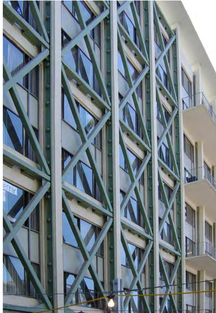
Structural retrofit to the exterior of building limits interior architectural impact.
