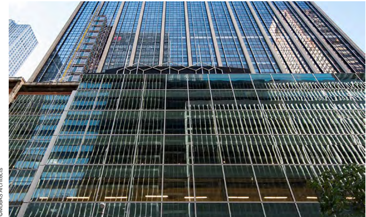
The re-cladding of this iconic 49-story tower from the 1950s allowed for deeper daylight penetration into workspaces, improving the wellbeing of building occupants. In addition, improvements to the façade and the performance of BMS systems yielded approximately 40% in energy savings and positioned the building to compete with newer high-rise offices.
