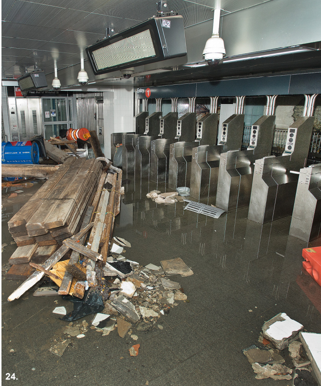
South Ferry subway station in New York was flooded during Hurricane Sandy
