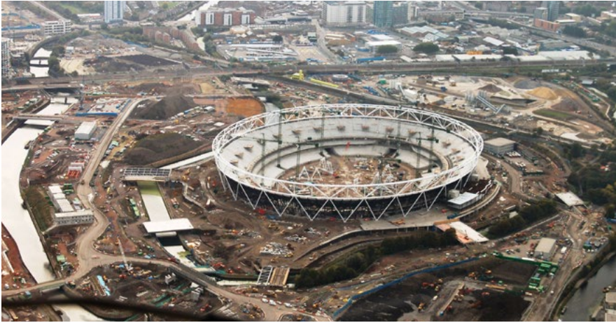
Olympic Stadium, Stratford, London: 98% of demolition material was reused or recycled
