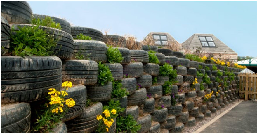
Dartington Primary School, UK: reclaimed tyres act as planters in the school grounds
