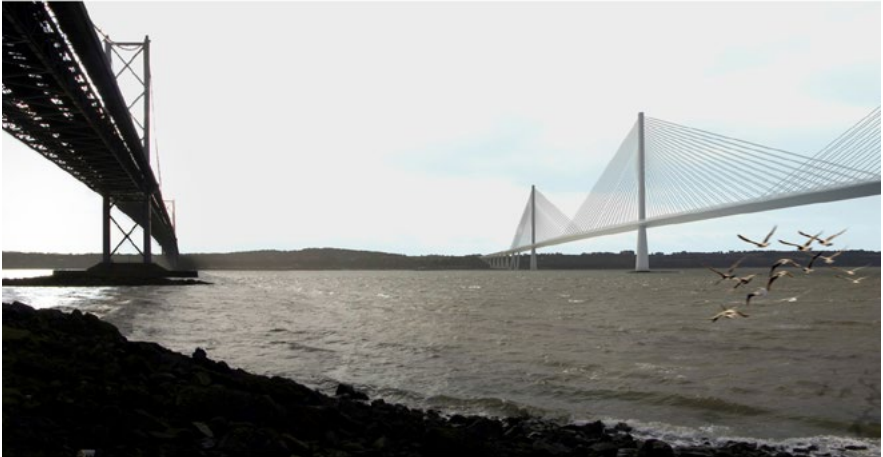
Scotland's Forth Replacement Crossing
