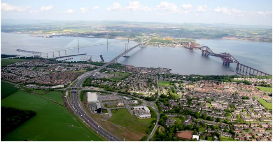
Scotland's Forth Replacement Crossing
