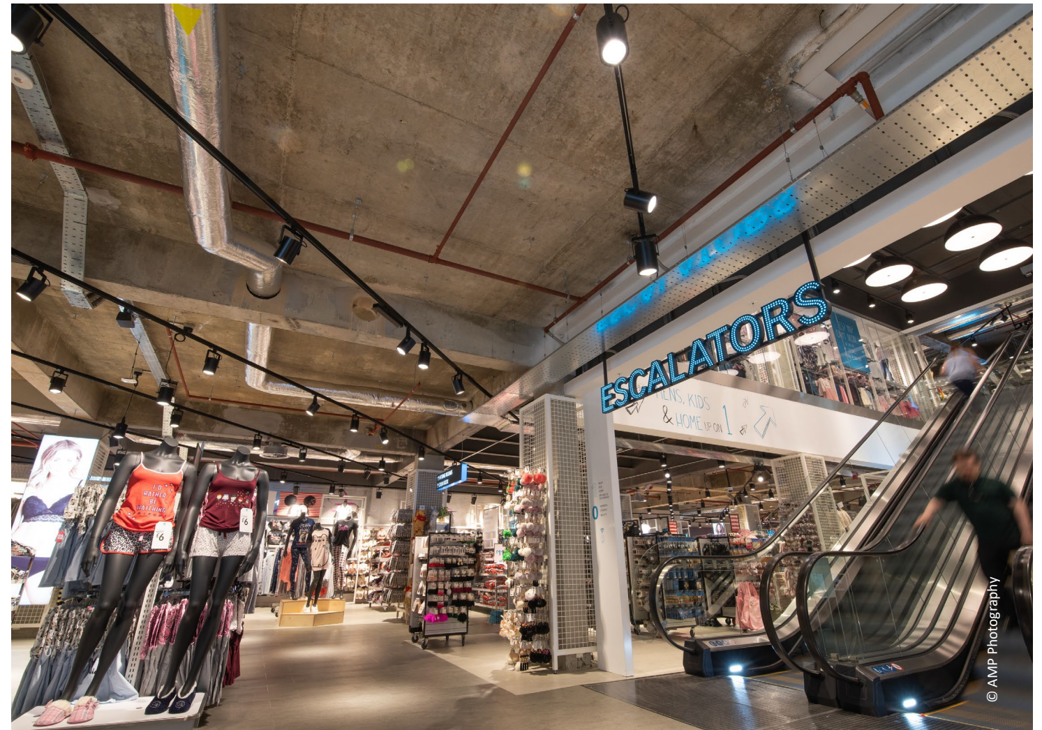
Repurposed existing buildings: 1960s reinforced concrete frame re-purposed into a modern, effective, large-scale department store
