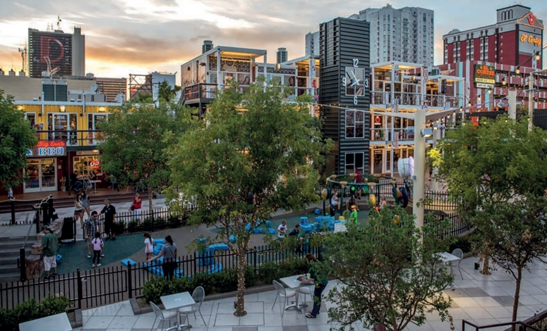
▲ Downtown Project in Las Vegas, USA
