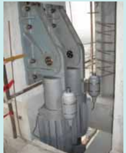
18. Both dampers in final position with pressure release valves fitted.
