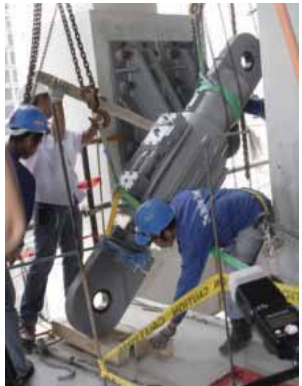
14. The dampers do not require special equipment to install.
