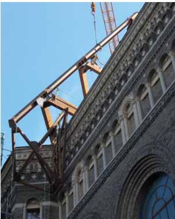
10. Crystal 5 overhanging the original building.
