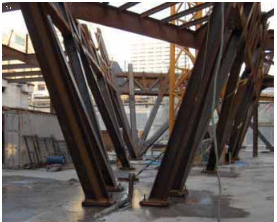
12. New frame adjacent to original building. 13. Crystal 5 spanning the original building. 14. Frame tailored to suit cladding arrangements. 15. Frame springing from "blockbuster" basement level.
