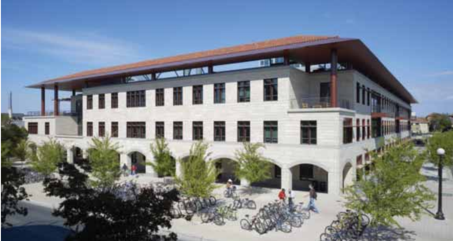
1. The west façade of the Jerry Yang and Akiko Yamazaki Environment and Energy Building.
