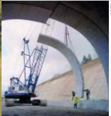
7. Eyhorne Tunnel arch being built.
