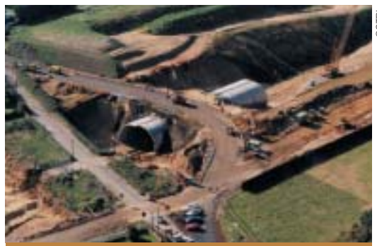
10. Sandway Tunnel precast arch.
