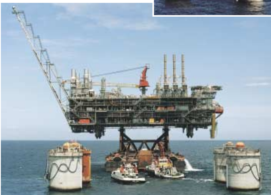
12. The topsides approaching the CGS for installation.
