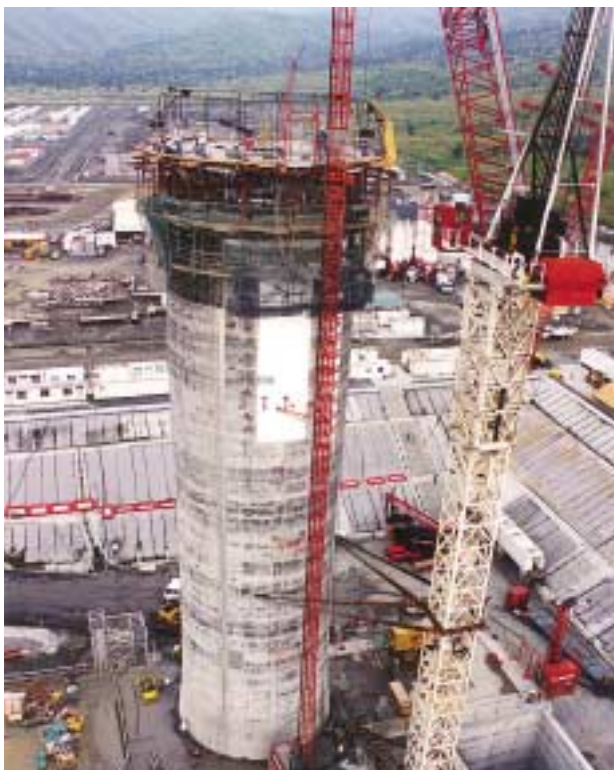
4. Utility shaft under construction, October 1999
