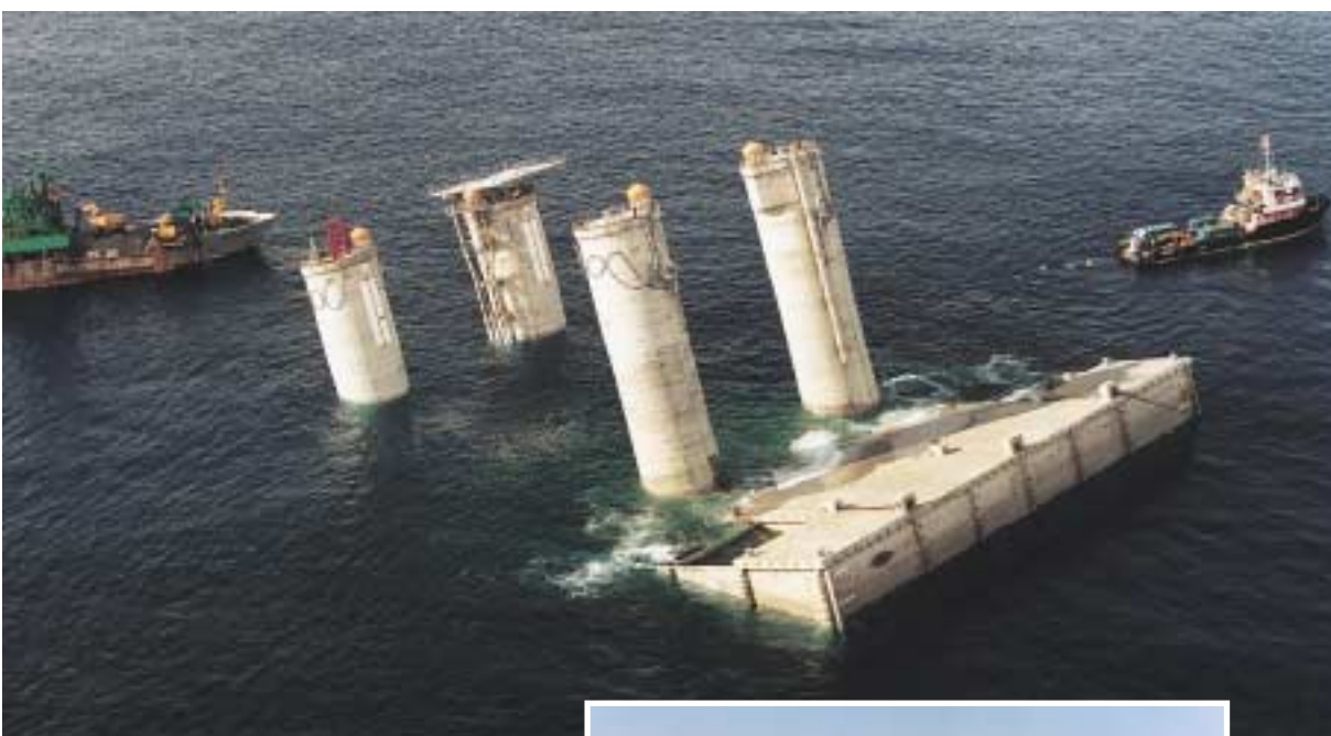
11. The CGS fully submerged in position awaiting topsides.
