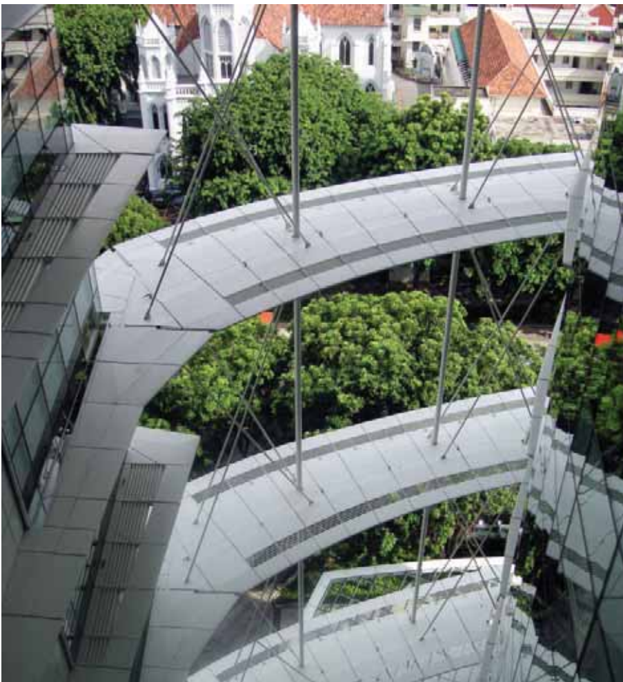
17. Sunshades in position in the laneway.
