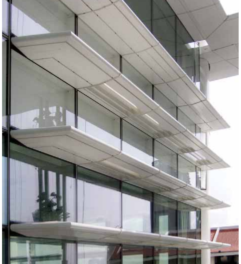
13. Exterior sunshades in place.
