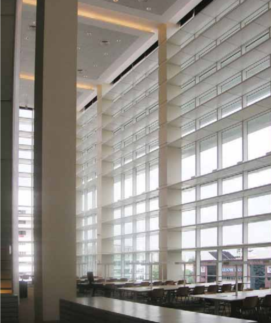
14. Interior sunshades in triple-height space.
