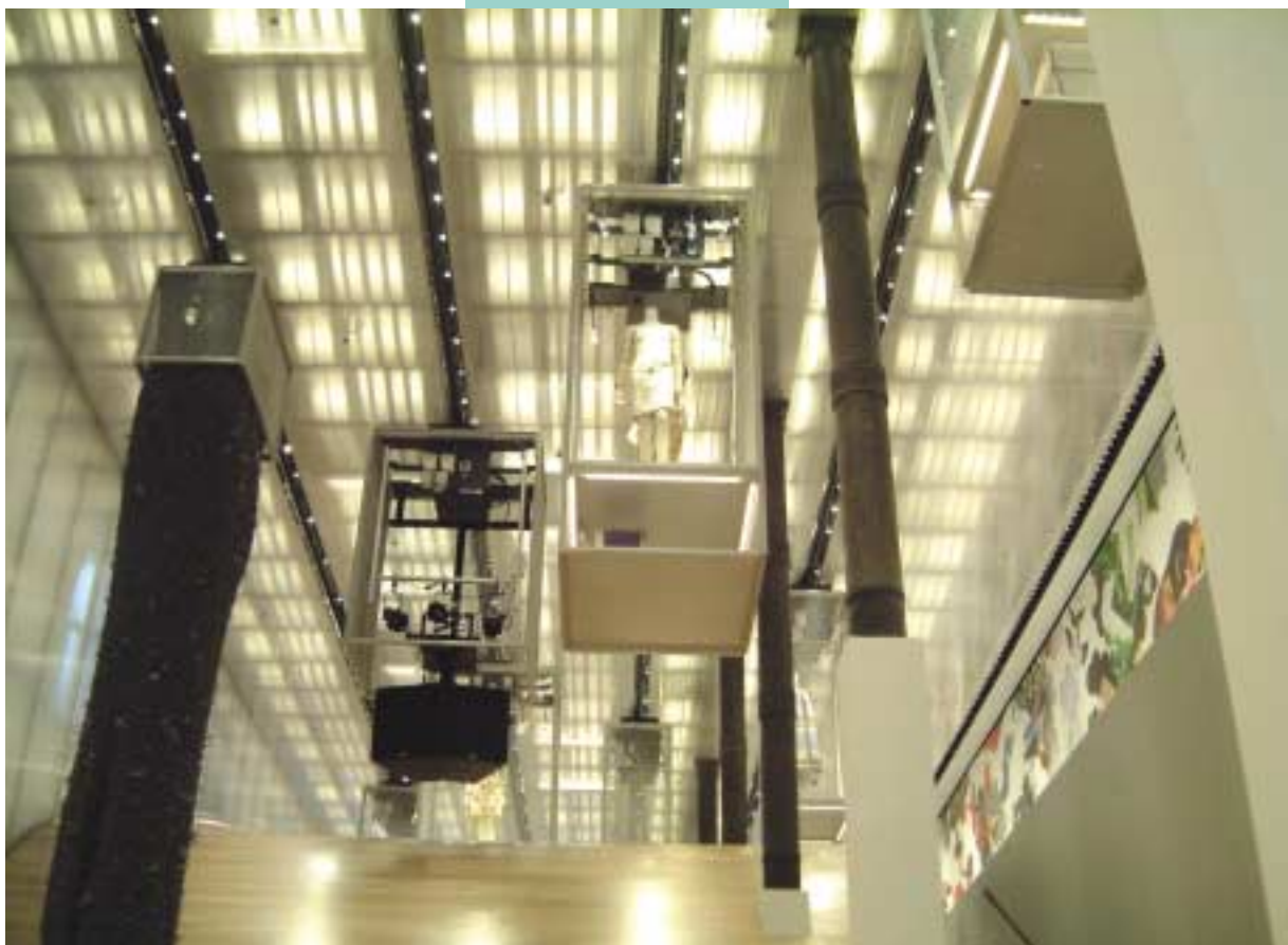
6:below: The movable, hanging volumes allow many space configurations. The crane system track and the cable raceways can be seen in the polycarbonate ceiling.
