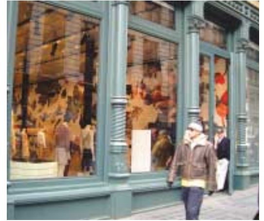
1. & 2. (right) The Broadway entrance: the original cast iron facade was retained while the interior of the store was completely re-worked.
