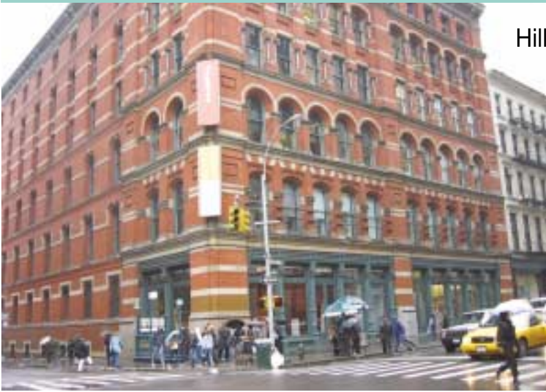
1. & 2. (right) The Broadway entrance: the original cast iron facade was retained while the interior of the store was completely re-worked.
