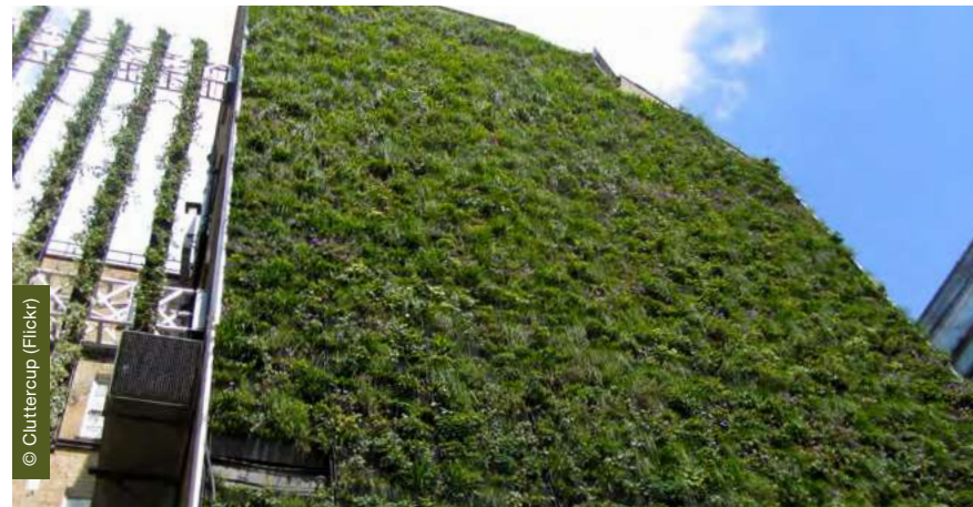
Green Wall, The Palace Hotel, London: Living walls can make a significant contribution to building cooling and insulation, thereby helping to lower energy consumption.
