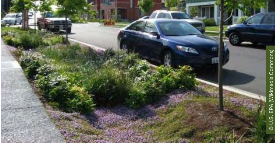
Road run off entering this sustainable drainage system in Seattle is cleaned by nature
