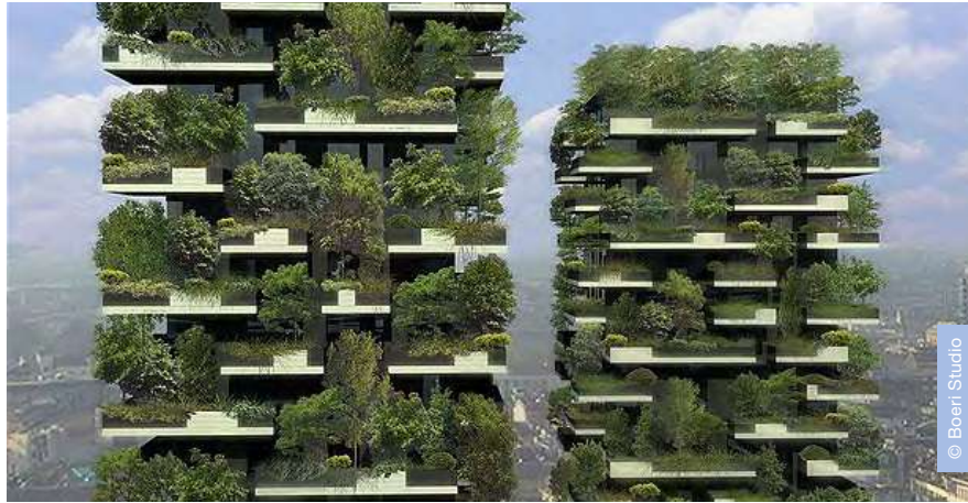
High-rise greening: The Bosco-verticale by Stefano Boeri, Milan. The concept is to reforest the inner cities with two high-rise apartment blocks covered with the maximum amount of vegetation.
