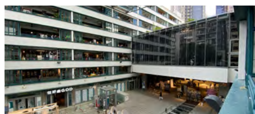
Sky-bridge connecting the two buildings
