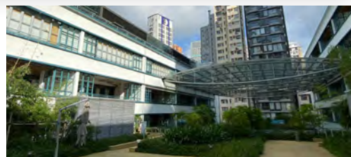
Roof garden on 4/F that is highly visible to visitors on both sides of the building
