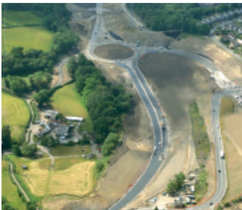
Aerial view of Church Village Bypass
