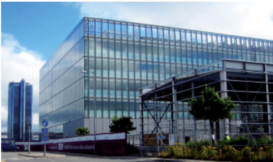
Above: BBC Scotland headquarters where Arup is providing extensive acoustics consultancy services
