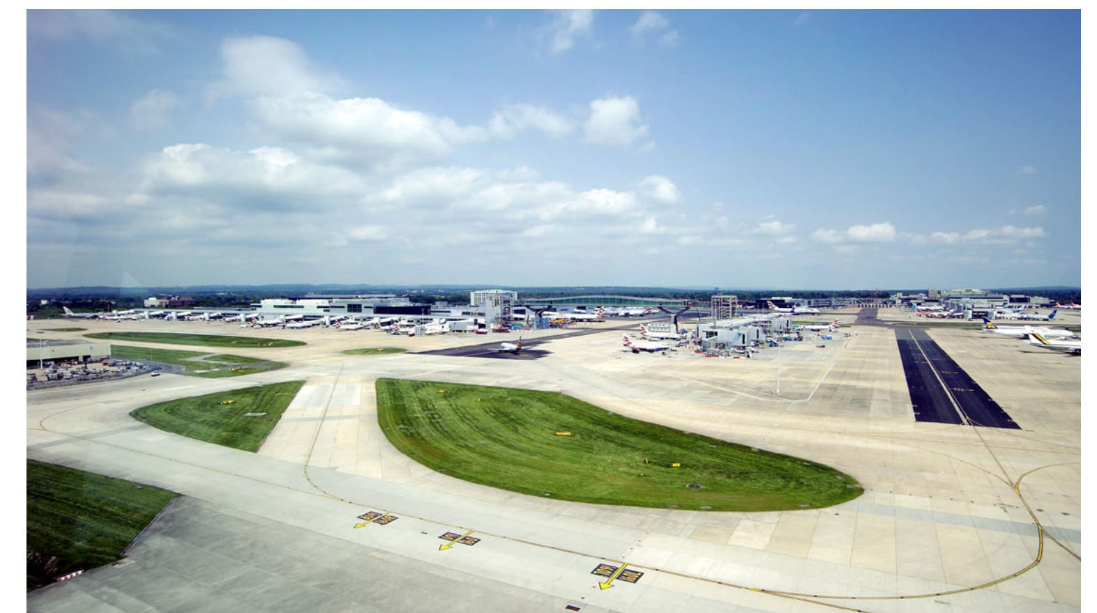
London Gatwick Airport Bridge, UK
