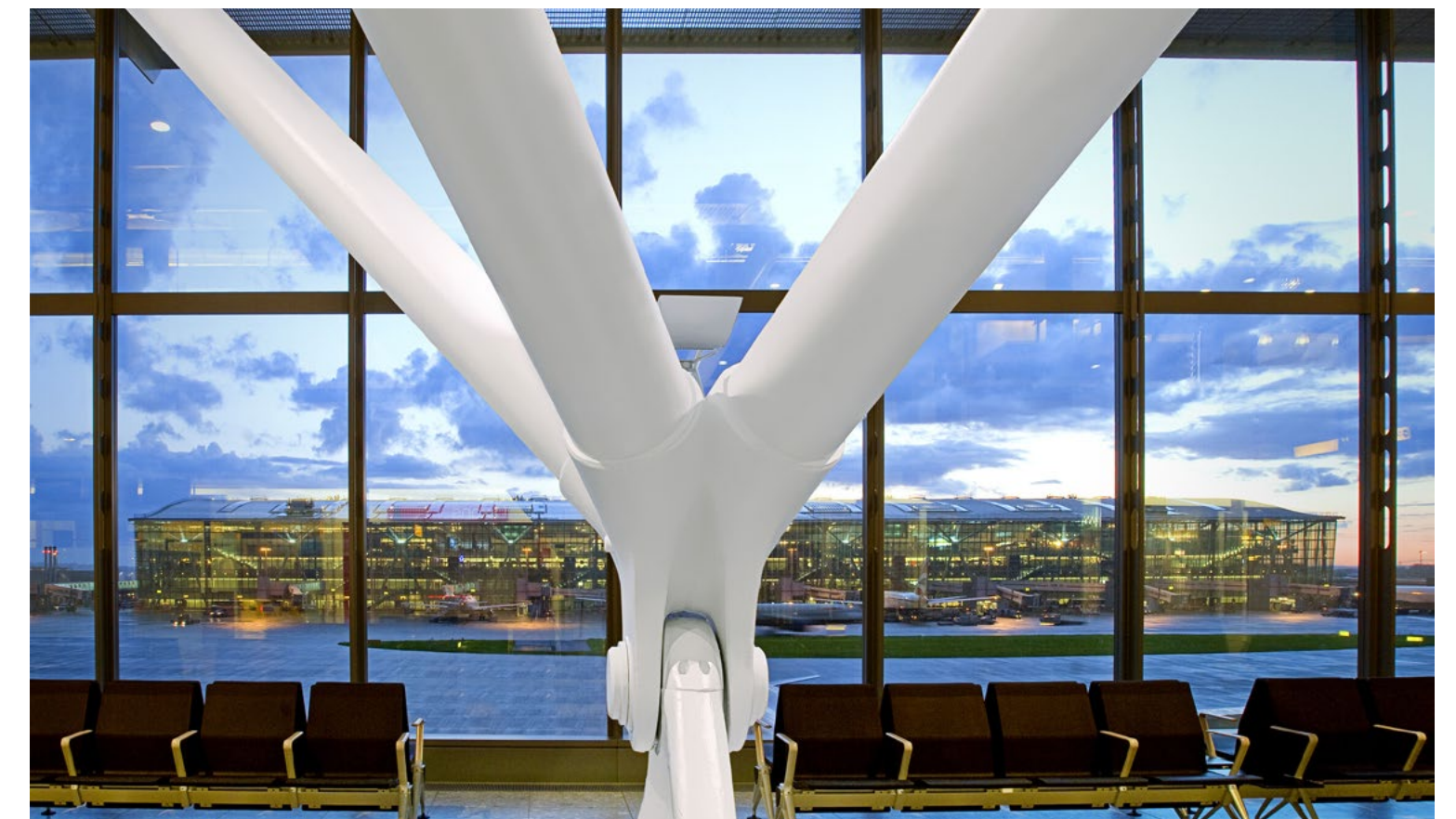
Terminal 5, London Heathrow Airport, UK
