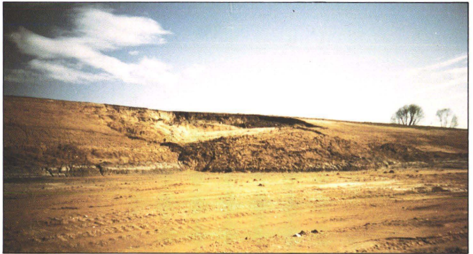
Above and below: Slope failure.
