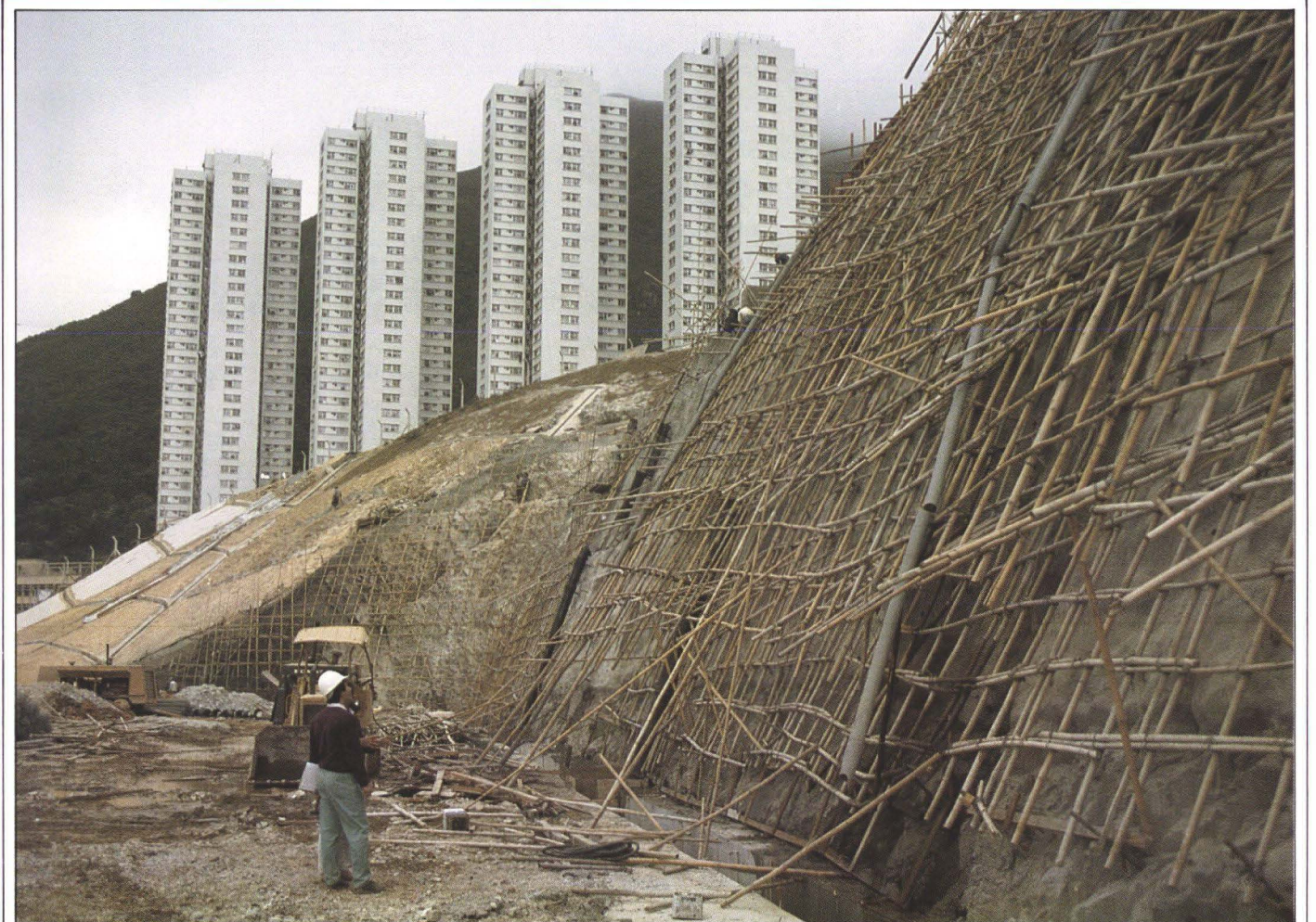
Hong Kong housing authority, slope remedial works (Photo: Martyn Stroud)
