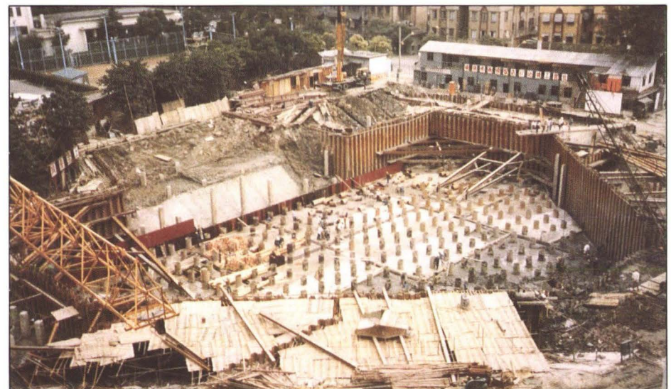
Jin Cang Mandarin Hotel: driven steel piles
