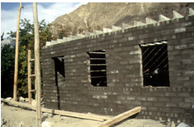
Figure 18. SELF HELP SCHOOL CONSTRUCTION PROGRAM, PAKISTAN. Guidance was issued on seismic construction detailing and site selection procedures.
