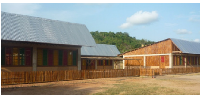
Figure 12b. SAFE SUSTAINABLE KINDERGARTEN SCHOOL MODEL, GHANA. A seismic hazard assessment for Ghana was undertaken to understand magnitude of seismic level the school needed to be designed for. Further analysis was undertaken to establish the most appropriate international code to be used for the seismic design analysis. The school was designed to meet Eurocode 8, the Earthquake design code.
