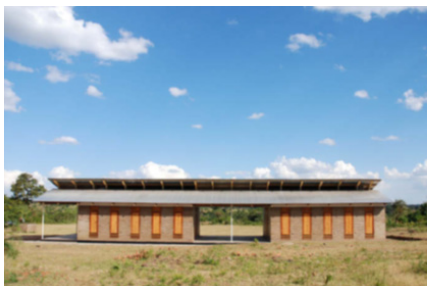
Figure 14. MALAWI SCHOOL PROTOTYPE. A low-cost, high performing primary school design for the Malawi Education Ministry to be rolled out throughout the country. The construction methodology was chosen to improve local construction practices specifically for seismic performance using locally available materials.
