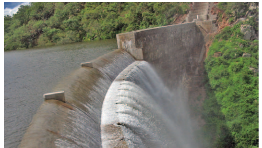
Large Dam Safety Inspections, Zimbabwe
