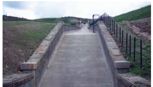
Windleden Reservoir, UK
