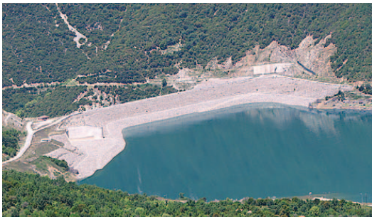
Evinos Dam, Greece
