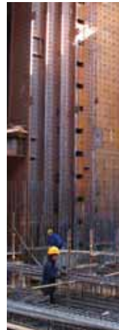
Left: The shaking table test. Above: The core structure. From the third level basement to the 16th storey, a unique steel plate shear wall was employed.
