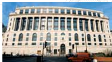
Restoring the iconic building (above) benefited from the early digging of deep caissons (below), which later helped to support the new internal structure (top).
