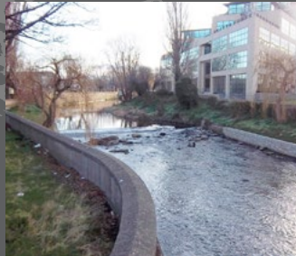
Dodder Flood Alleviation Works, Dublin, Ireland
