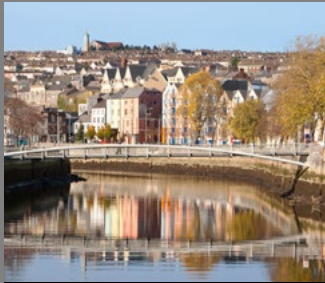
Lower Lee Flood Alleviation Works, Cork, Ireland
