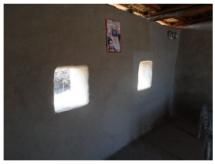
Acceptability – The shelter had good thermal mass with multiple openings resulting in good internal environment which was light and ventilated. However it was scored down on security as no windows or doors were provided. The shelter programme was integrated and no consideration was made for cooking and WATSAN.
