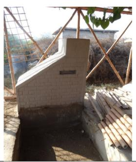
Photo 10 Heritage Foundation, Tando Allah Yar Full scale section through an adobe brick foundation for training purposes
