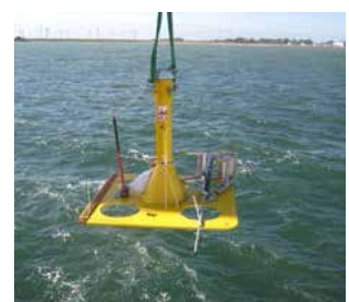
Installation of referencing device for pile testing.
