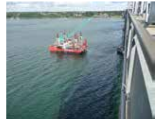
Jack Up Drilling Platform in Lillebaelt
