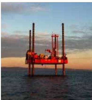
Transfer to Jack-up
