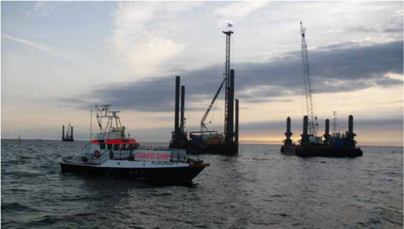
Numerous Jack-ups and Guard Vessels in Femern Strait
