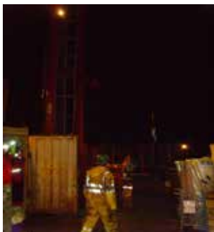
Supervising Night Drilling Operations
