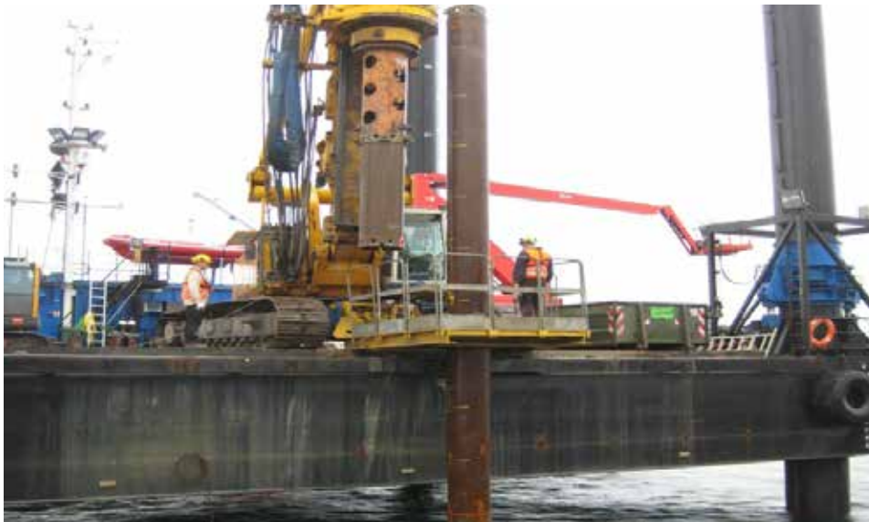
Installation of Driven Piles
