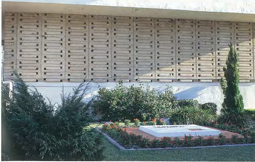
5. Annie Pfeiffer Chapel is constructed of structural reinforced concrete with 'textile' block infill walls.
