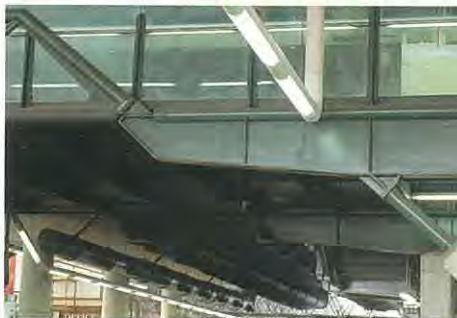
6. Cantilevered main beam on Mezzanine Bridge.
