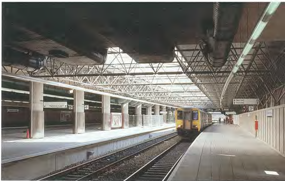
5. Platforms 3 and 4 west, with new canopy and exhaust ventilation systems above.
