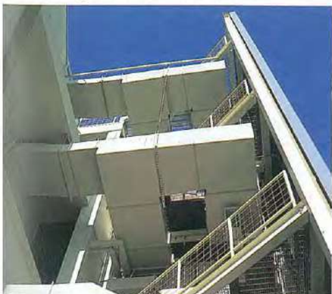
Paramount archive: 8. Horizontal ductwork and piping distribution. 9. Level-by-level mechanical distribution.
