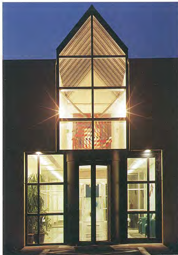
7. Entrance to the administration building.
