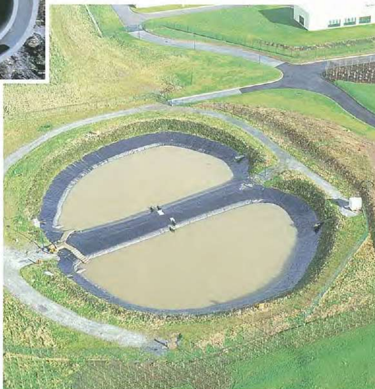
12. Completed retention pond: this acts as a catch basin for all storm/fire-water run-off.
