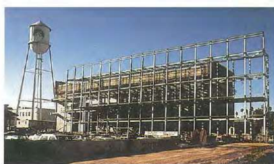
2. Paramount archive under construction.
