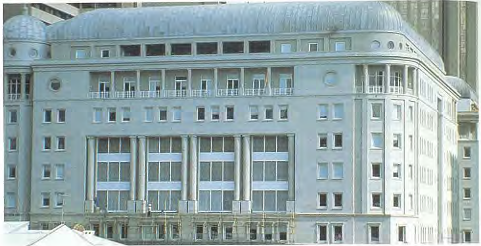
9. Completed building. The façade utilises Paarl and Rustenburg granite in preference to the Naboomspruit Sandstone originally favoured.
