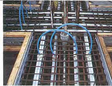
6. Post-tensioned beams: intersection detail.
