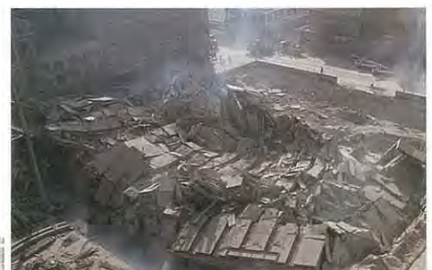
7. Collapsed buildings following implosion.
