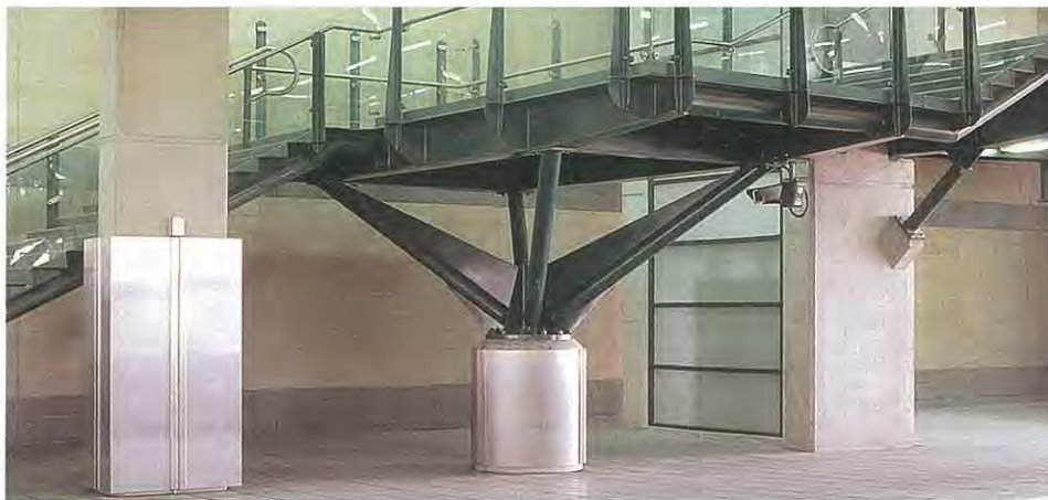
7. Mezzanine Bridge: stair landing support detail.
