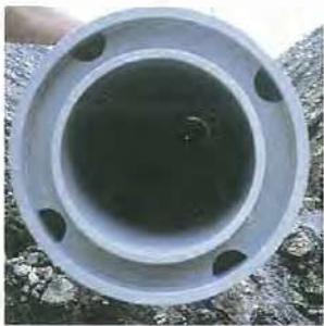
11. Section through polypropylene process sewer.
