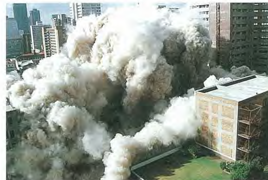
6. Five buildings demolished by one implosion.
