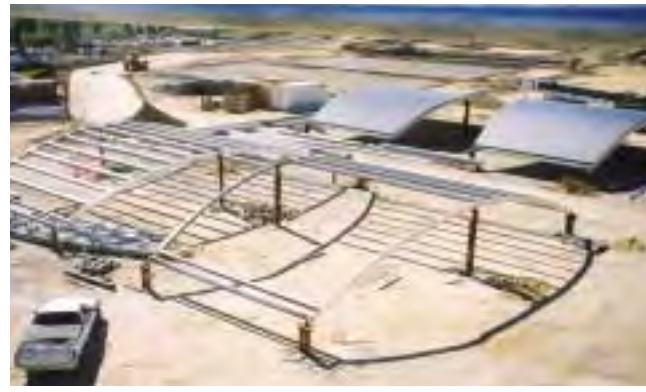
11. Roof panel prefabrication.
