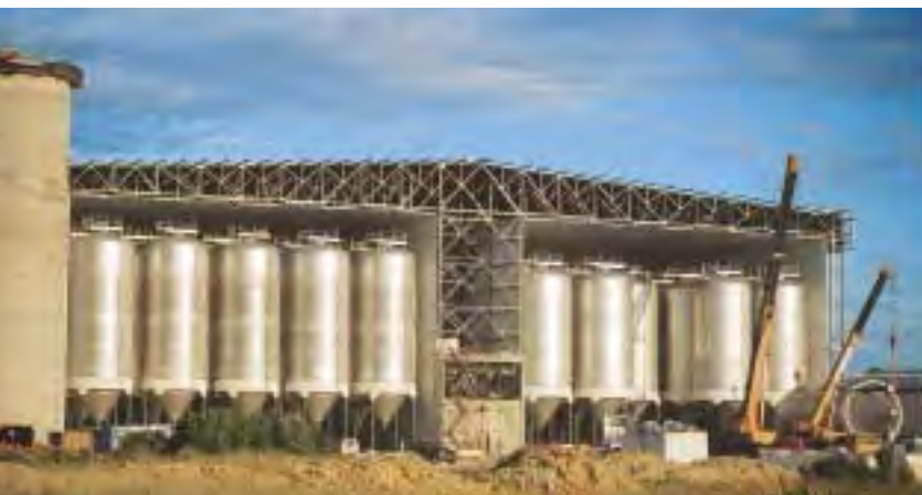
6. Cellar building at completion of tank installation.
