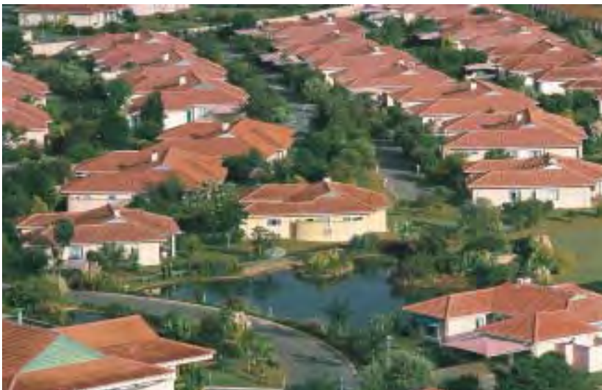
3. Foreground left: access road crossing the irrigation storage pond, behind the community centre.
