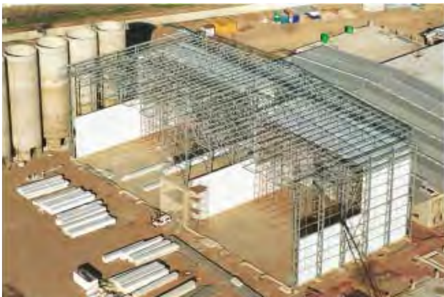
7. Cellar structure's insulated paneling partially completed.
