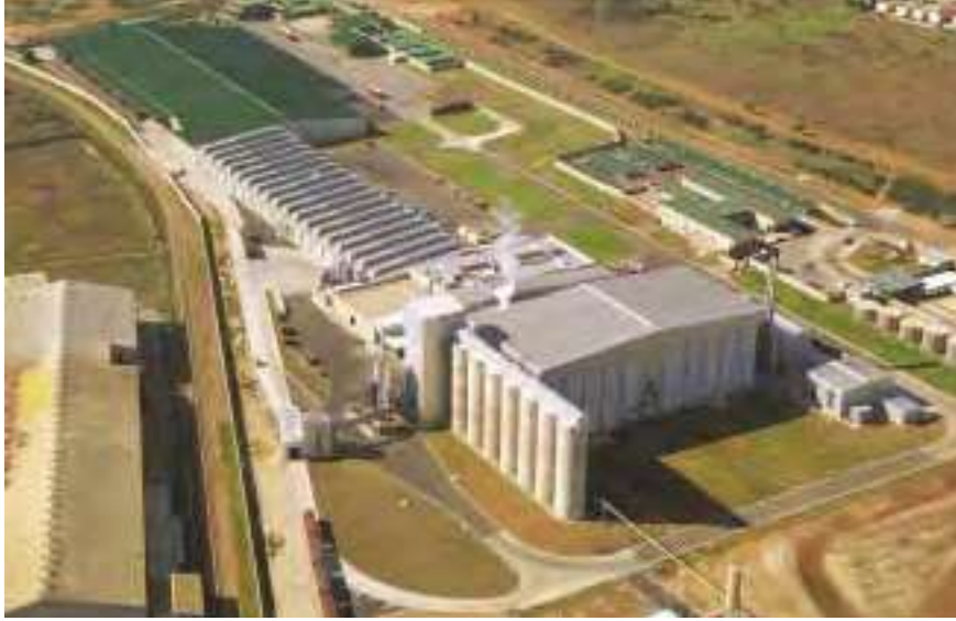
5. SAB Ibhayi Brewery from the north-west.
