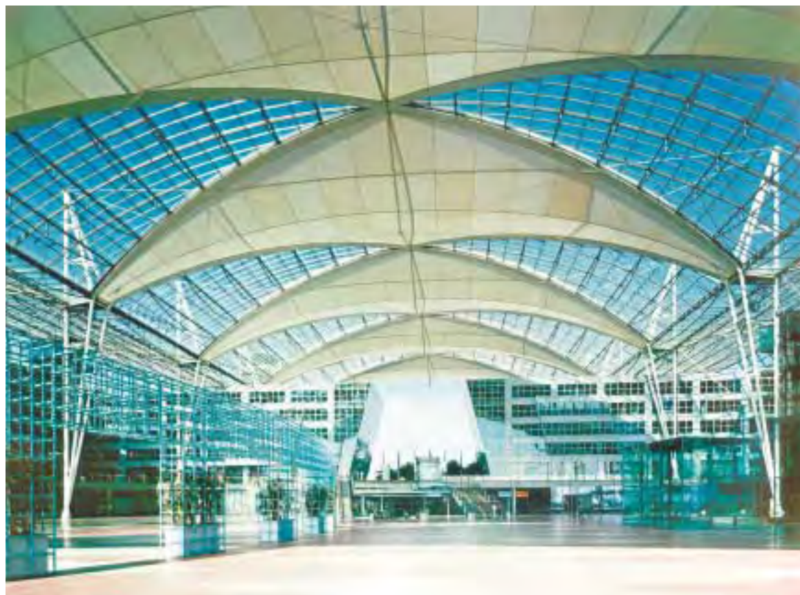
9. The roof seen from the Forum space along the central axis; the main entry platform is at the far end.
