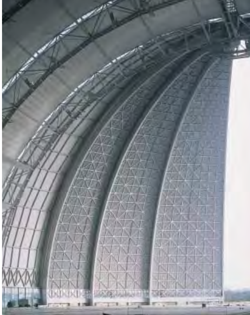
14. On opening, the door segments nest inside each other.
