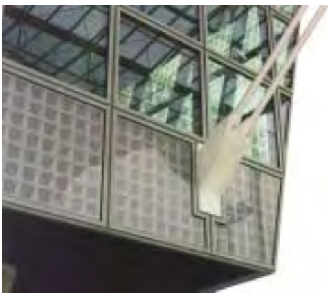
6. Backstay connection to building.
