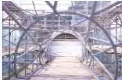
4. Tubular sleeve and alternating rods in place.
