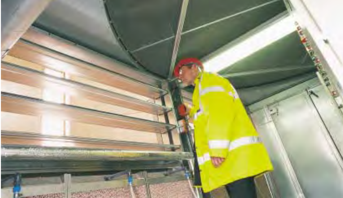
9. Interior of lower part of AHU, with engineer beneath thermal wheel, looking through bypass damper.
