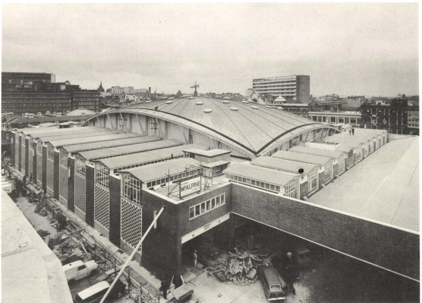
Above: Smithfield Market interior. Below: An exterior view. The shell is an elliptical paraboloid 230ft x 130ft.
