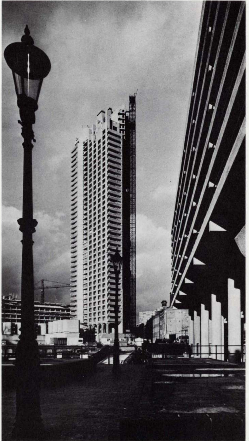
Fig. 66 Barbican Redevelopment Scheme, London Architects: Chamberlin, Powell & Bon
