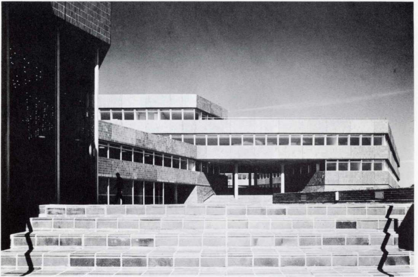
Fig. 63 Sunderland Civic Centre Architects: Sir Basil Spence, Bonnington & Collins Completed: 1970
