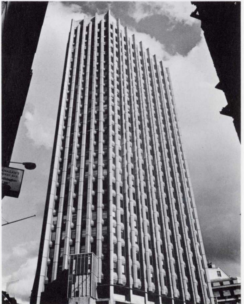
Fig. 64 The Stock Exchange London Architects: Llewelyn-Davies, Weeks, Forestier-Walker & Bor and Fitzroy Robinson & Partners Completed: 1970 (Phase A)
