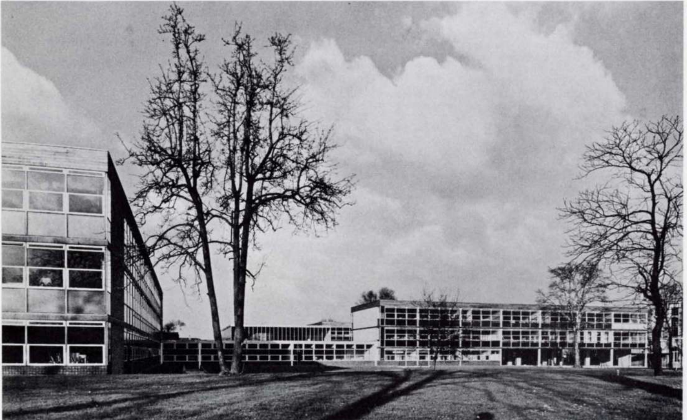
Fig. 9 Cement and Concrete Association, Research Laboratories, Wexham Springs, Bucks. Architect: W. R. Oram Completed: 1956
