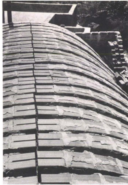
Fig. 4c Cullinans : 4.5m span lounge (Photo : Ove Arup & Partners, Zimbabwe)
