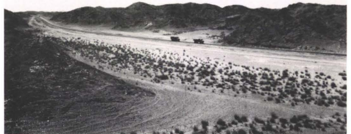
Fig. 3 Existing road through wadi in igneous rock terrain (Photo: Keith Law)
