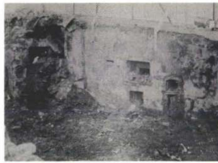
Fig. 4 Basement wall exposed during construction
