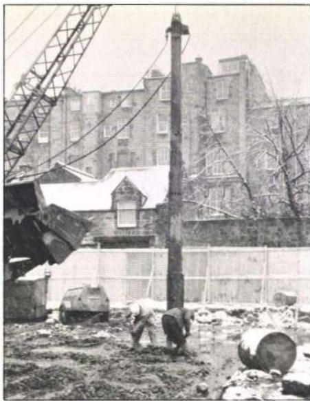
Fig. 7 Vibroflat in operation at the site (Photo: Ove Arup Partnership)
