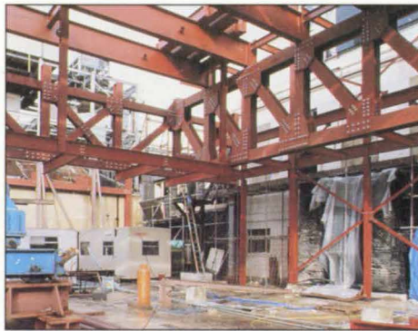
7. Steelwork transfer girders for cineplex.
