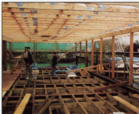
1. The new timber frame under construction.
