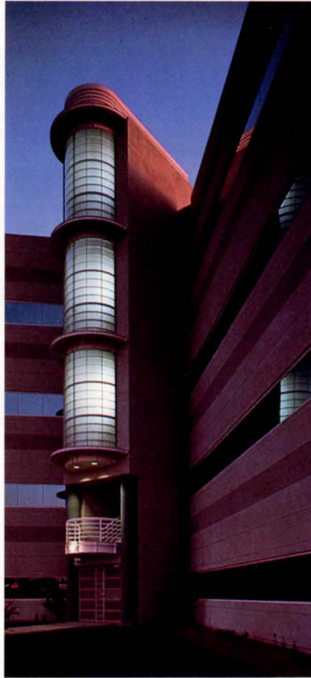
3. Phase 1 MOB from interior courtyard, looking north.
