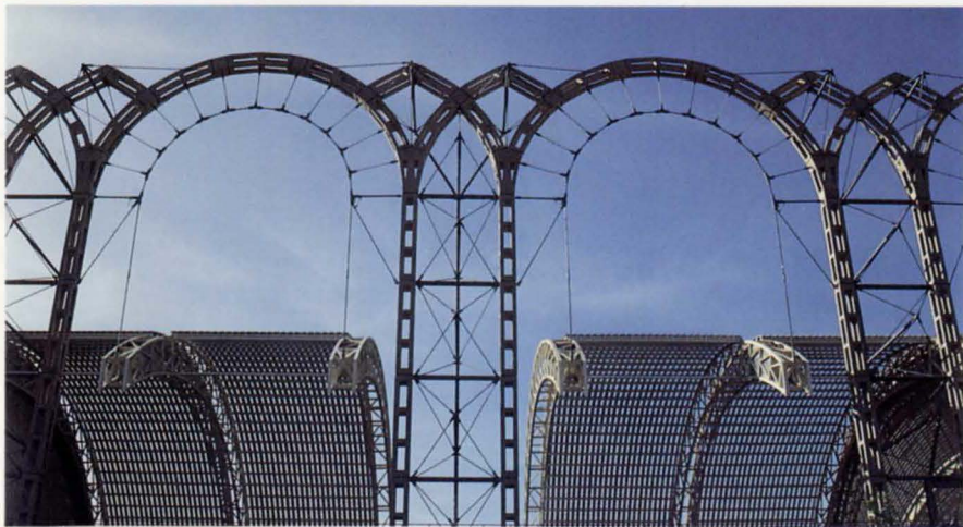
7. The stone arches of the Pavilion of the Future for Expo '92 in Seville, Spain. Similar to a web, the lightness of the structure is achieved by designing for deflections rather than preventing them.
