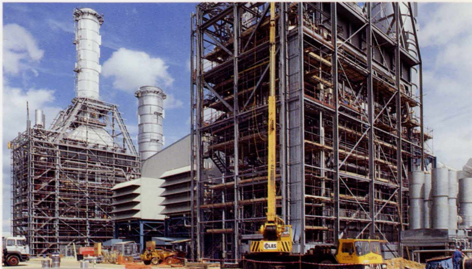
14. Peterborough heat recovery boilers under construction.
