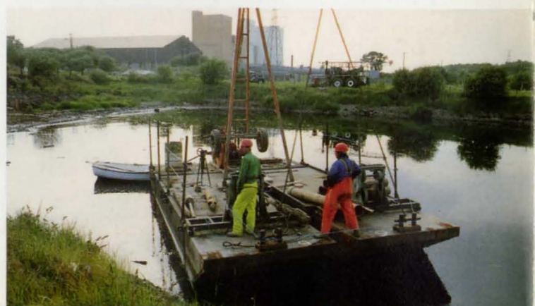
9. Corby ponds before reclamation: pontoon and drilling rig on pond 2 during the site investigation.
