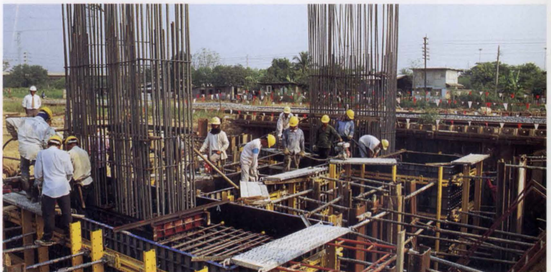
8. Pilecap construction.
