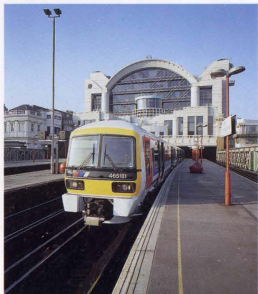
1. Class 465 entering Charing Cross beneath Embankment Place (also an Arup project).
