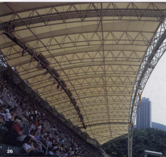
5. Catwalks on underside of roof structure.
