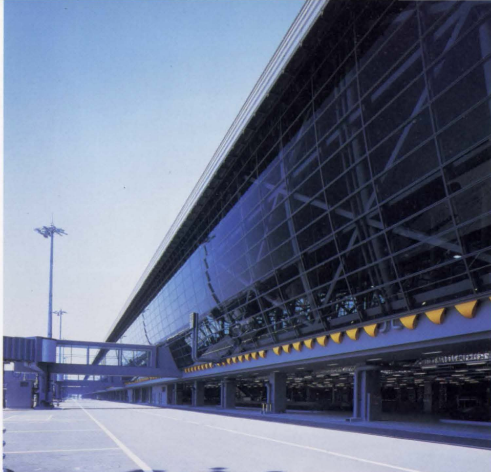
13. 'Fish tail' ducts supply air to Wing.
