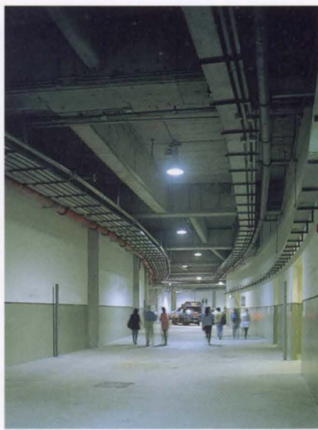
3. Access driveway for goods vehicles.
