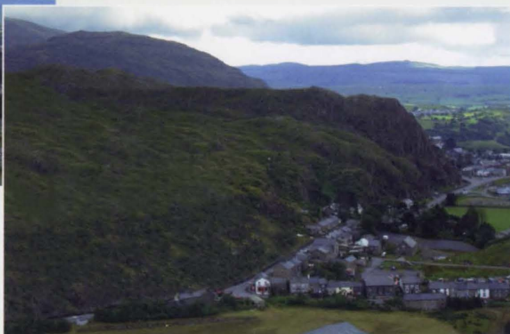
b. As it could appear, after removal of slate tips and restoration work.
