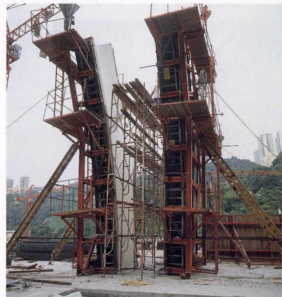
8. Wooden formwork on steel subframes used in achieving the exposed concrete finish on raking beams.
