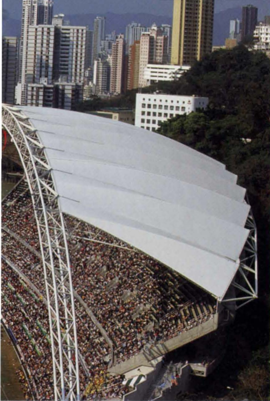
9. The fabric roof.
