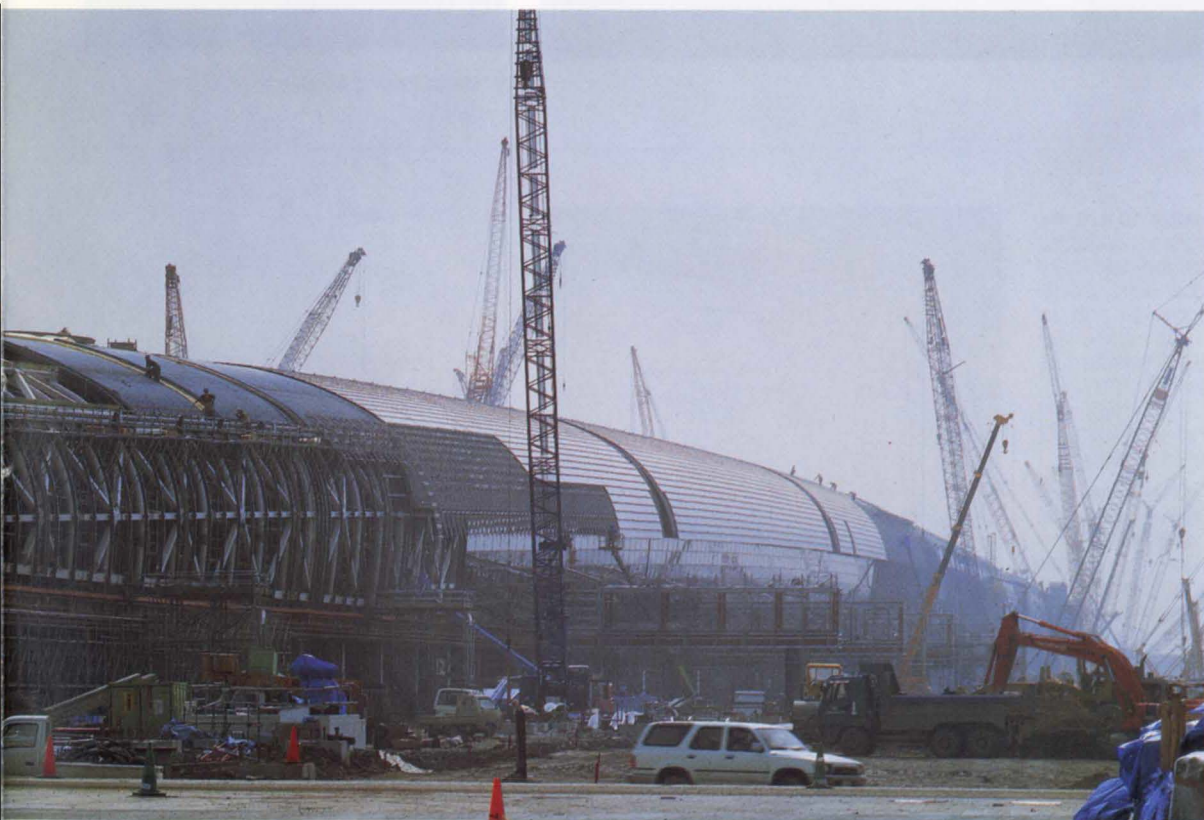
10. Wing under construction, August 1993.
