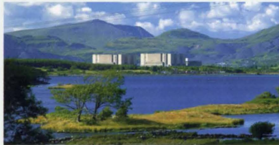
b. The reactor buildings lowered to c.30m.
