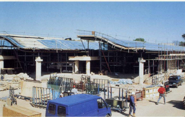
12. Construction work in progress.
