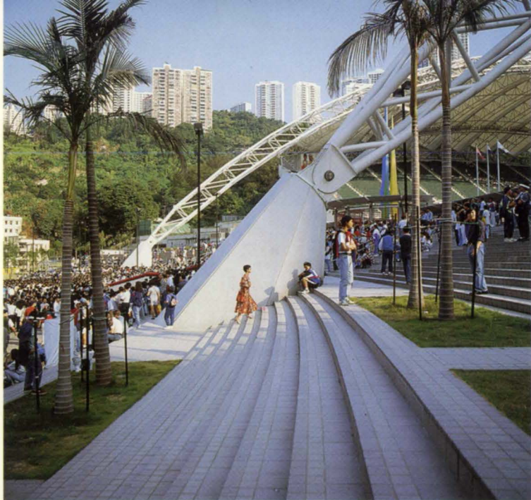
15. View of roof truss bearing and abutment.
