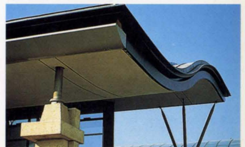
10. Detail of roof corner support.
