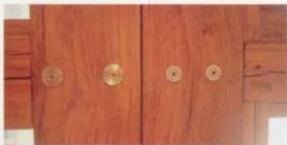
3. Window-frame joint detail.
