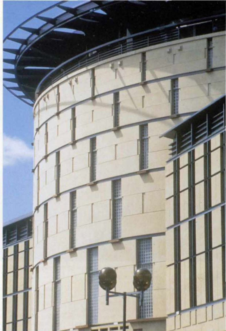
13. Above: Precast units on exterior of the drum.
