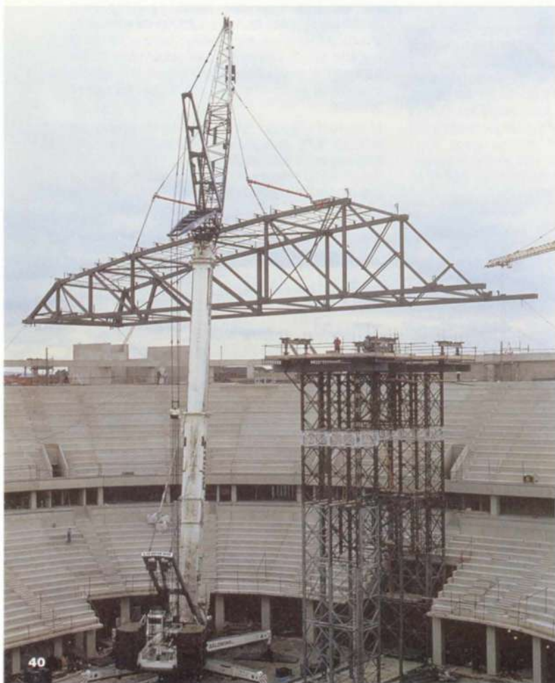
8. Roof truss lift.
