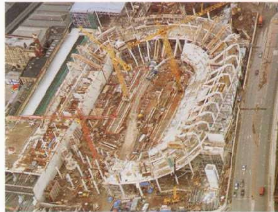
6. Arena concrete frame under construction.
