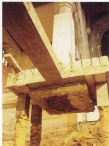
9. Underside of pier.
