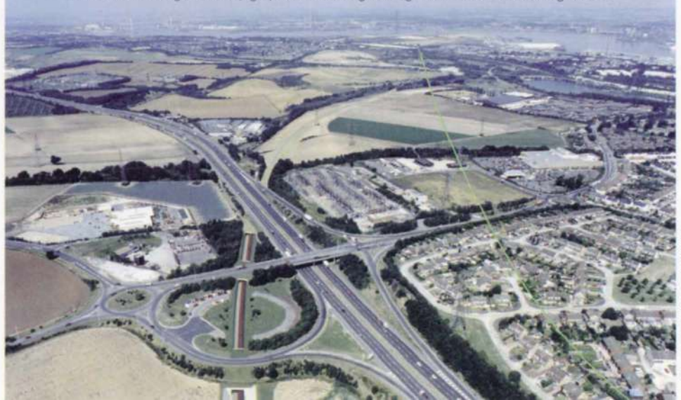
1. Pepper Hill: This superimposition shows the final route (left) in a cut-and-cover tunnel under the A2/B2175 intersection. The green line (right) shows the original alignment under the housing estate.
