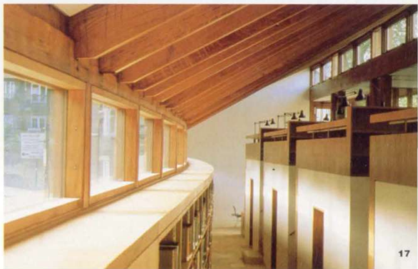
7. Pitched roof beams.
