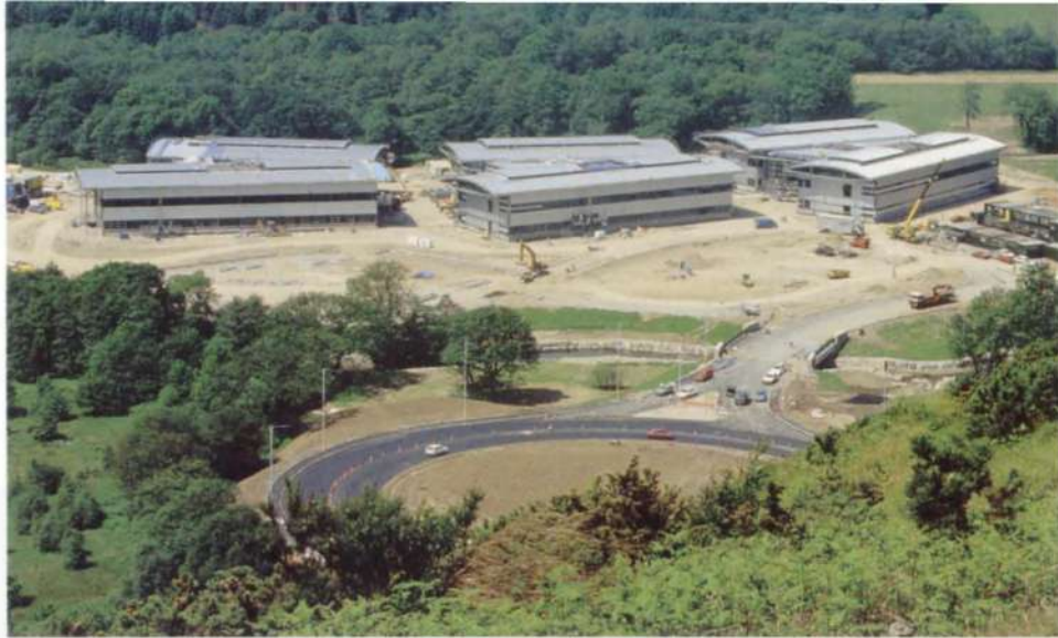
1. The site during construction.
