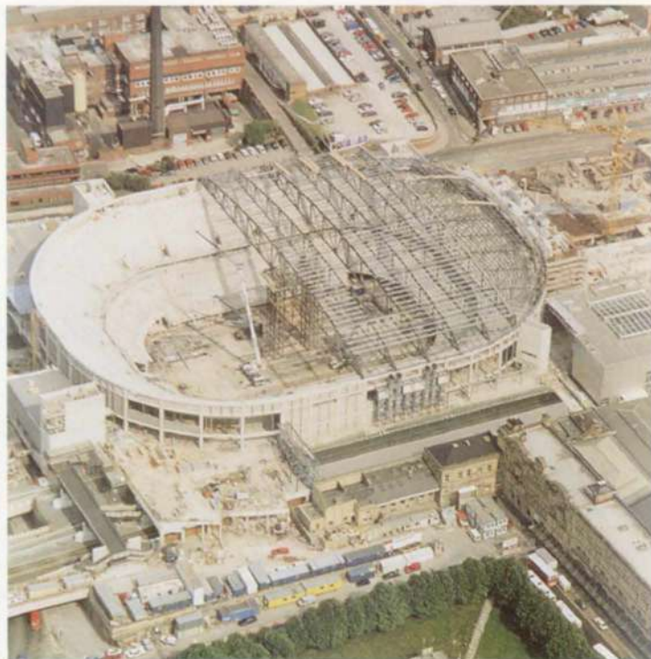
9. Below: Concrete frame almost complete with half of roof steelwork erected.
