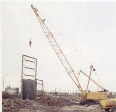
5. Lowering HDPE membrane into wall.
