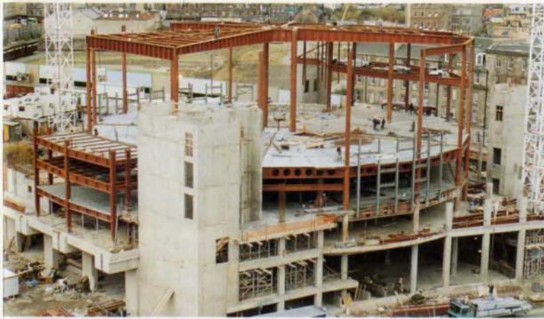
11. Progress on site by November 1993, showing the steel structure of the auditorium drum:
