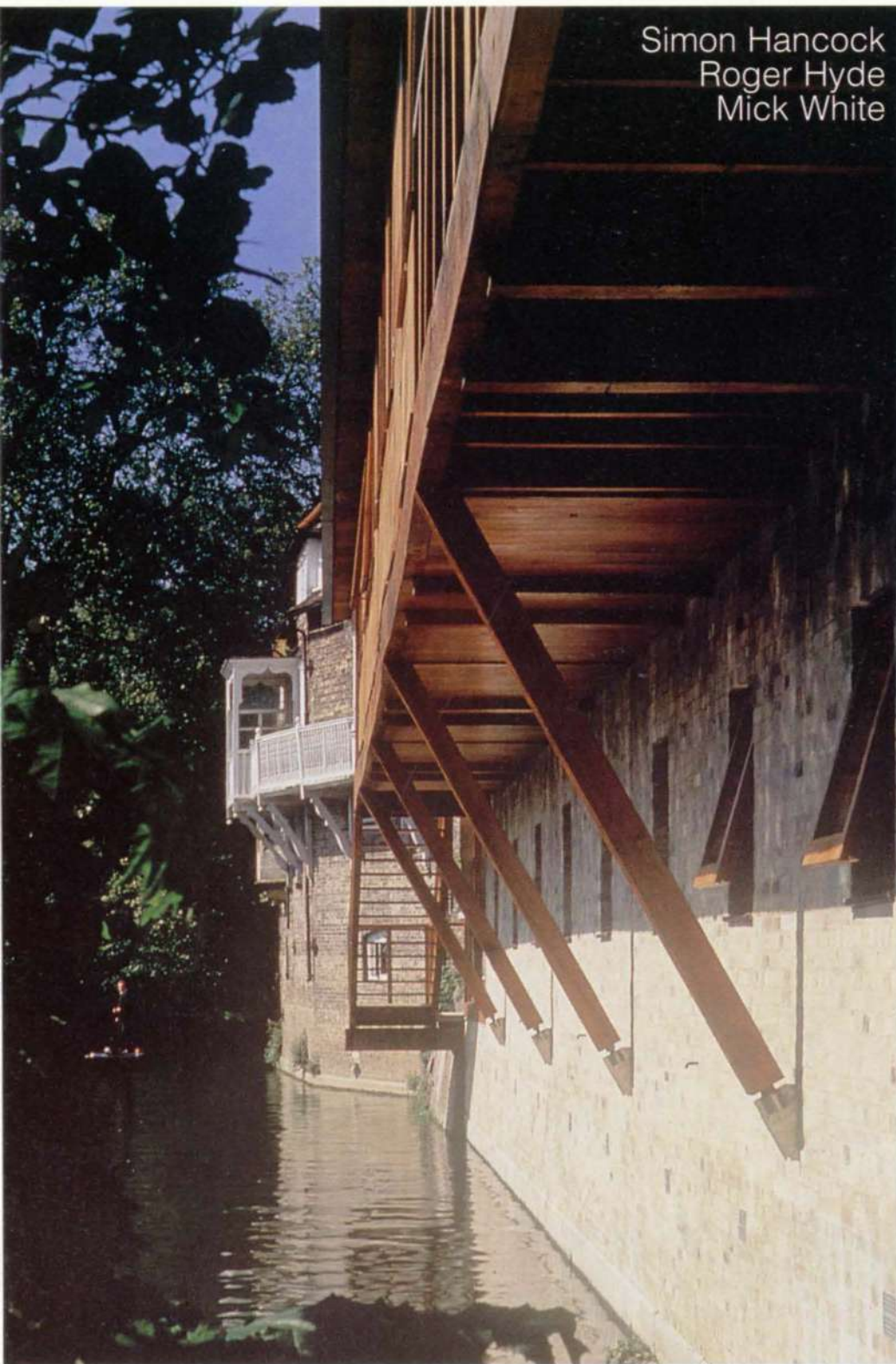
1. Darwin College: Oak beams support the cantilevered study area over the River.
