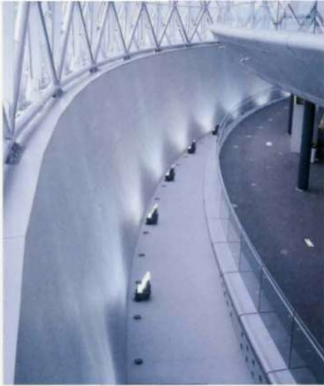
13 above: Inside the dome perimeter, showing the space between the dome and the internal floors..
