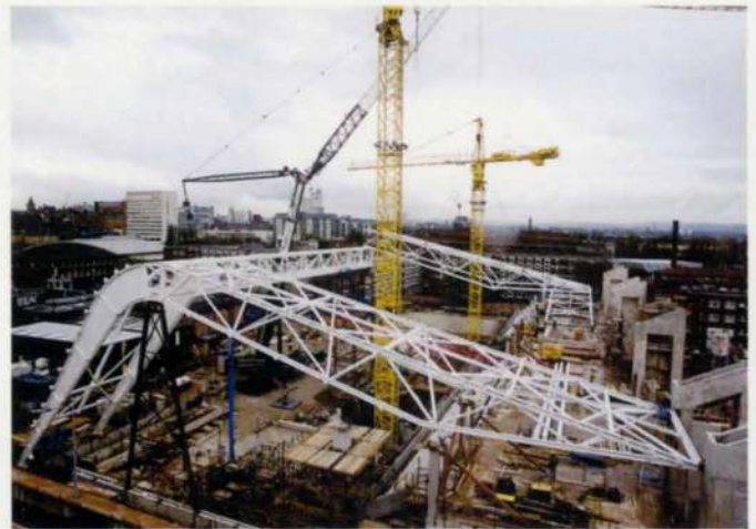
5. Craning in a complete pair of main ribs.
