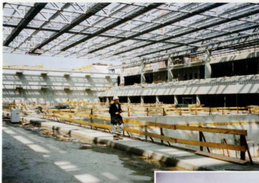
6. Partially launched Schwimmhalle roof.
