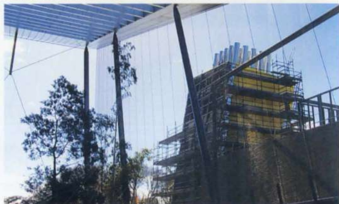
9. One corner of the Forest Gallery, showing cable-supported mesh enclosure and its degree of transparency.
