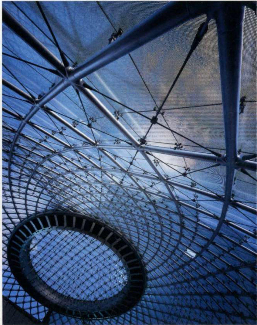
15. The diagrid shell and the ring beam.
