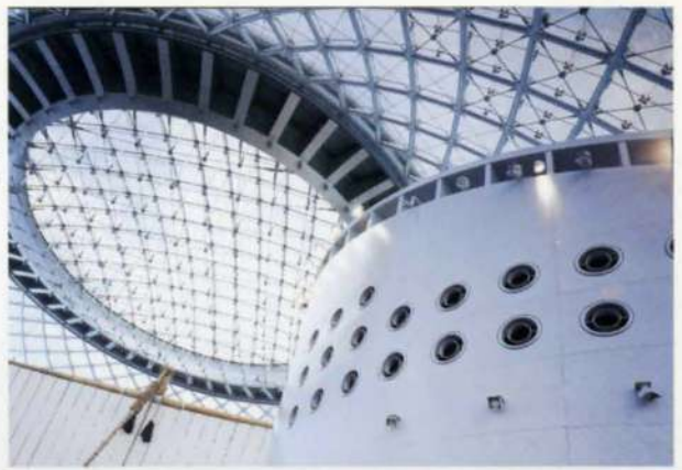
14. Close up of ring beam and core structure (note ventilation ducts on the wall)
