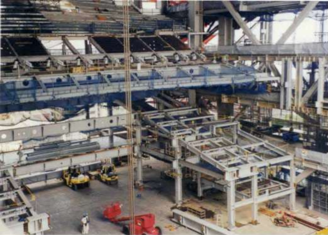
17. The auditorium under construction.
