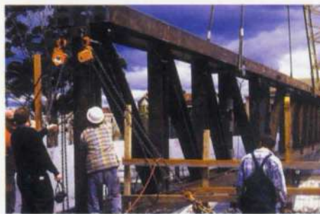
15. IMAX theatre transfer truss ST3 being lowered into position.
