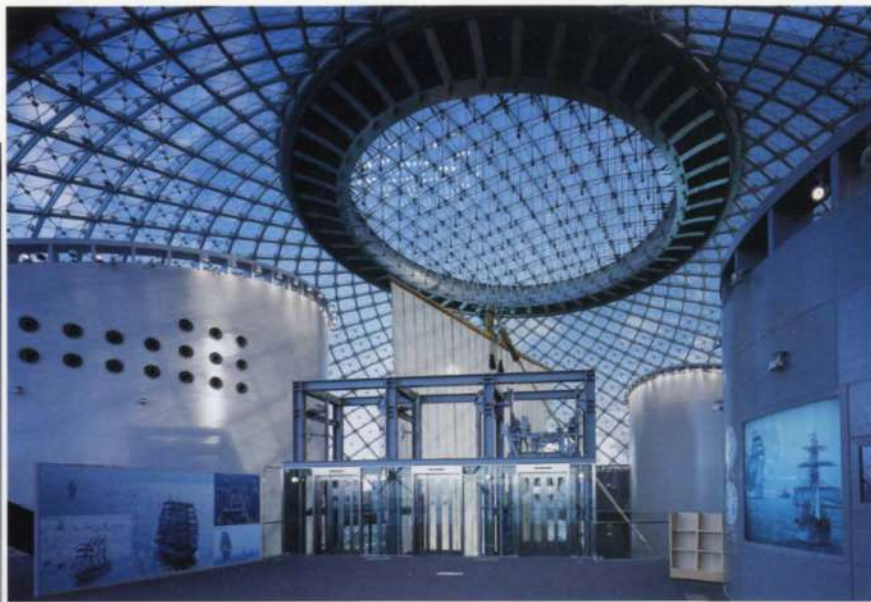
10. The third floor, showing the three core structures, the transparent riser, and the ring beam above.
