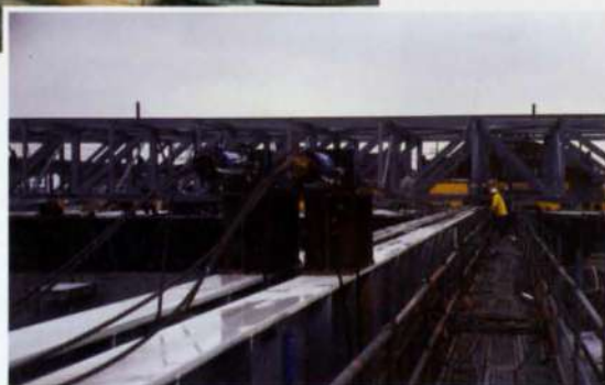
7. Launch rails and jacking point.
