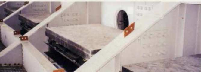
19. Tuned mass dampers.
