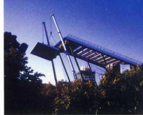
16. Cantilevered tip of Forest Gallery canopy being dual crane lifted into position.
