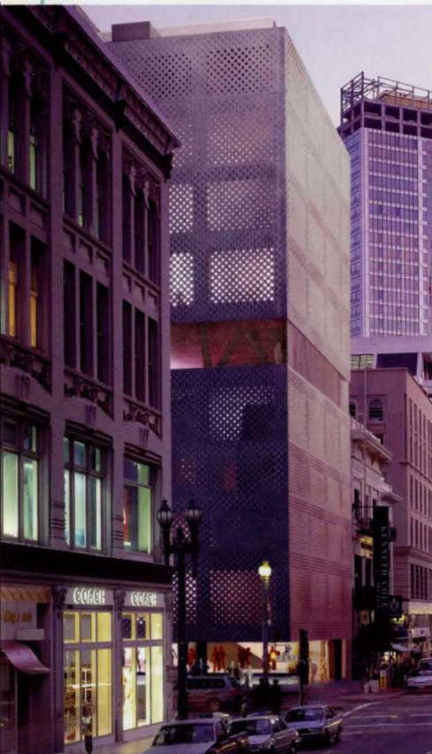
9. San Francisco: a 10-storey flagship store providing 37 000ft 2 (3440m 2 ) of retail and office space with a unique structural system of base isolation and perforated steel shear panels to resist lateral forces.
