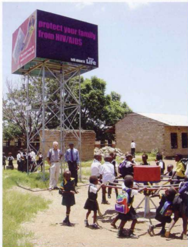
6. Children at play turning a roundabout bolted above an existing borehole. This action works a pump enabling drinking water to be pumped into an overhead storage tank screened with billboards promoting HIV/AIDS awareness to the community.
