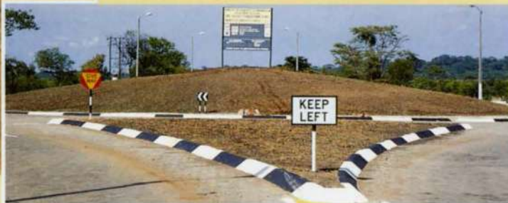
4. Roundabout crossing with main Harare/Bulawayo road raised centrally to prevent glare from oncoming vehicles. This requires street lights for 24-hour operation.
