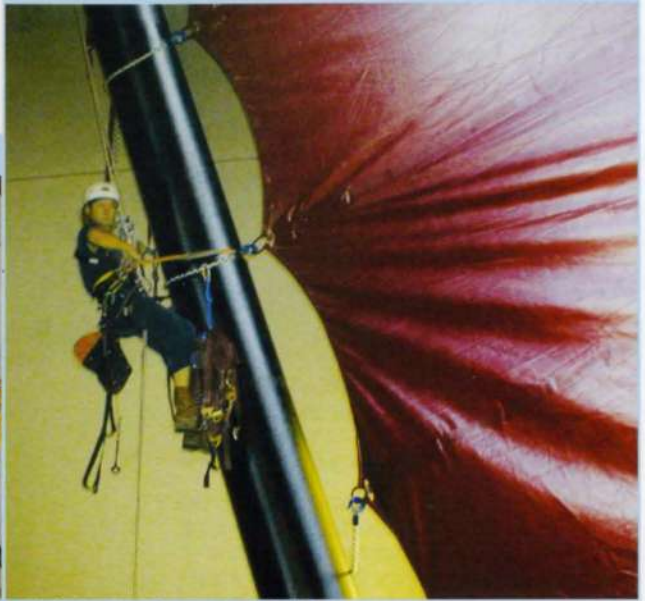
9. Abseiler securing connection
