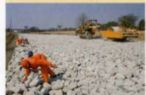
10. Compacting rock fill layer and hand screening of oversized rocks.
