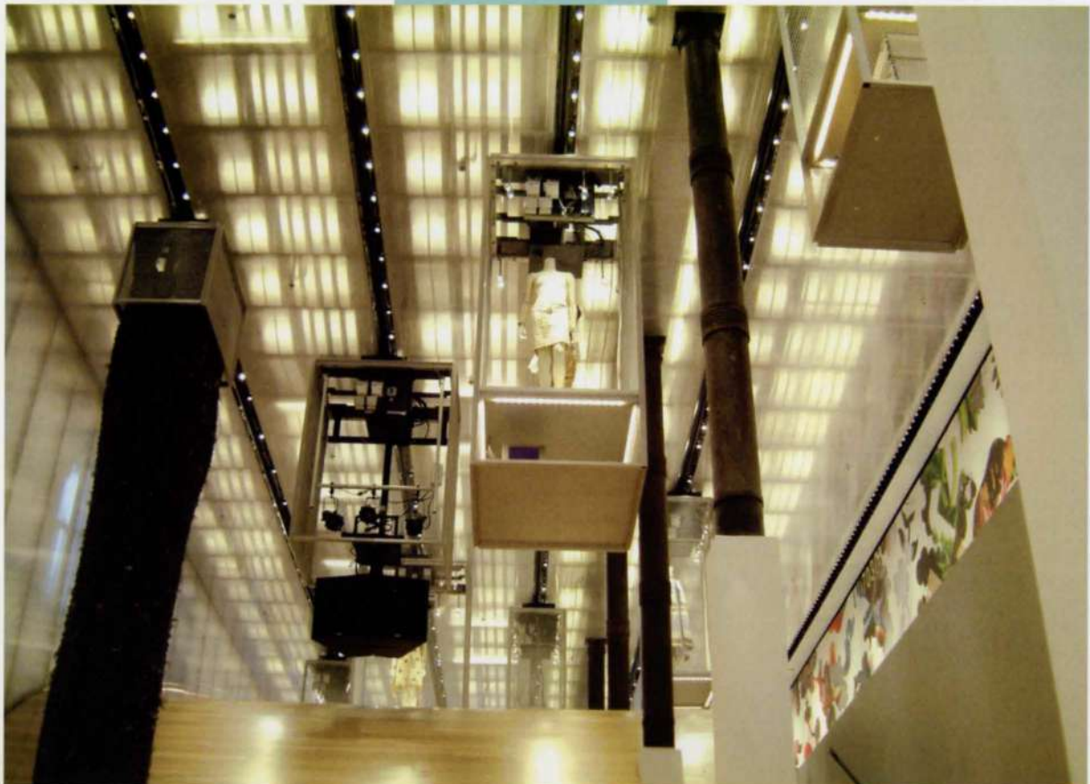
8 below: The movable, hanging volumes allow many space configurations. The crane system track and the cable runways can be seen in the polycarbonate ceiling.
