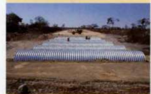
8. Six-bore Armco multiple culvert.
