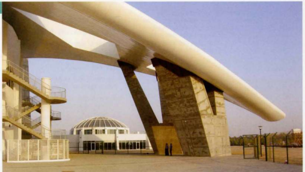
5. One of the concrete abutments to the roof.
