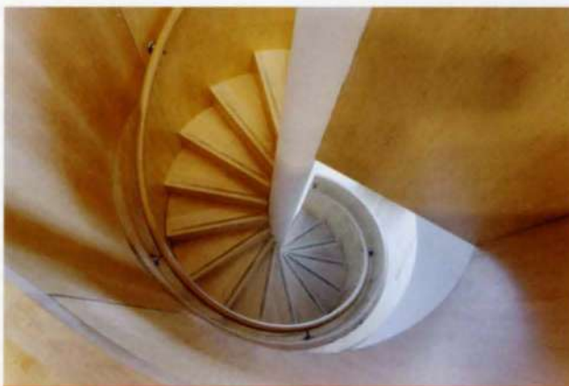
8. Internal staircase: economy of space.
