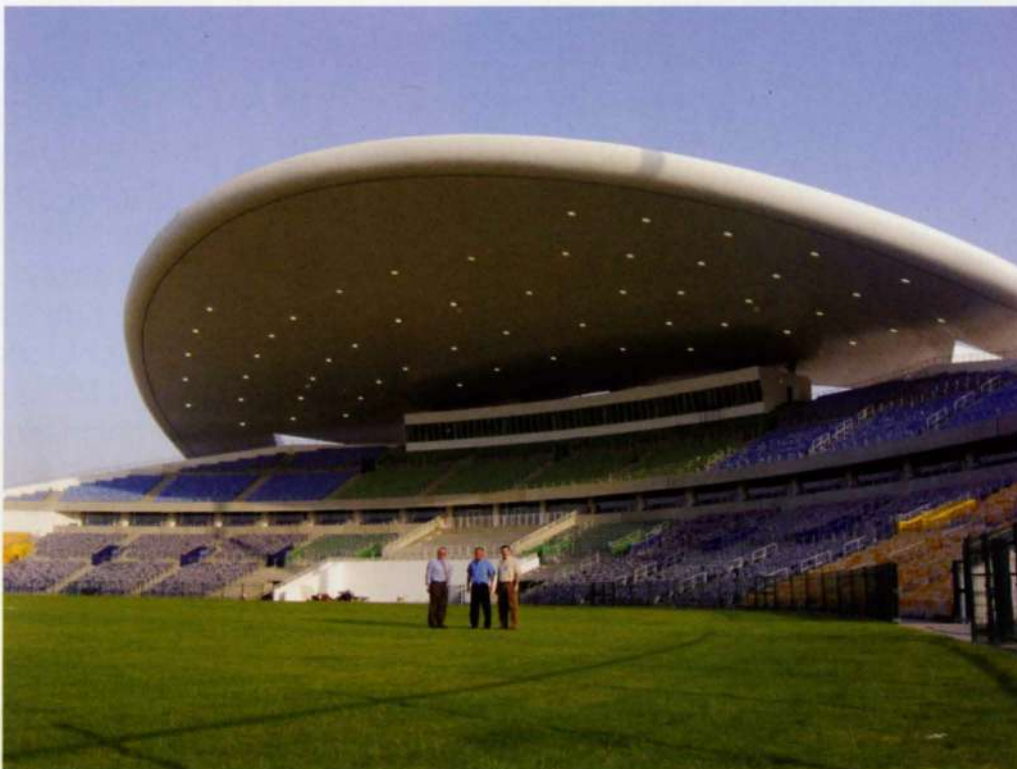
7. The completed roof in position.
