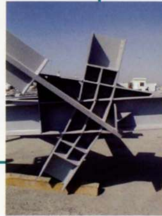
6. Truss intersection node.
