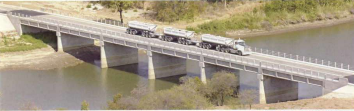
12. Mupfure River Bridge: 112m long with precast concrete beams and cast in situ slab. This method cost more than the traditional cast in situ beam and slab, but was faster and did not require staging in the potentially flooded river bed.
