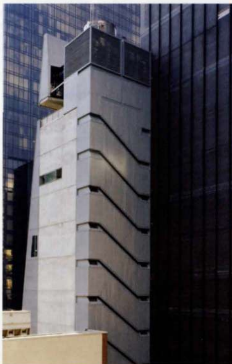
9. Staircase with water tower above, ventilation louvre at each side, and cooling tower louvred enclosure.
