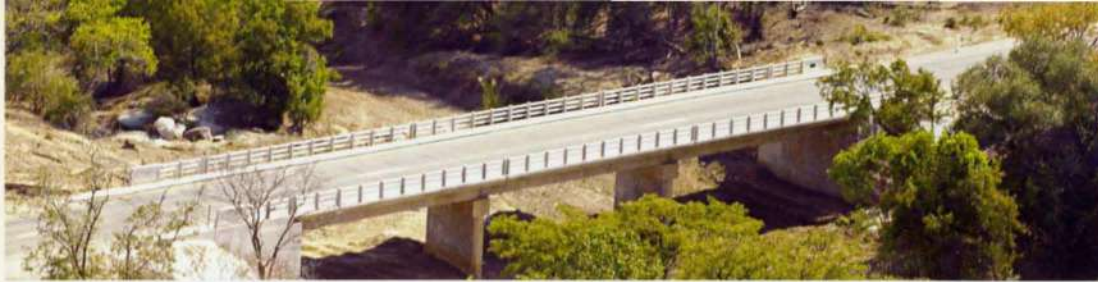
6. Seruwe River Bridge: 36m long, cast in situ solid slab deck.
