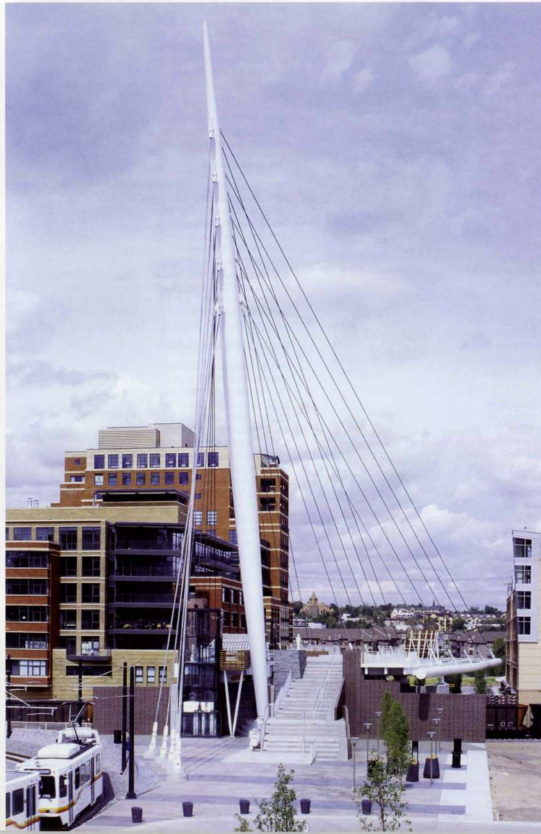
8. The bridge viewed from the city.
