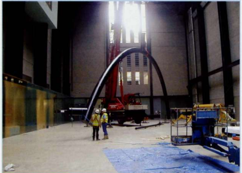
7. Commencing erection of east steel ring.
