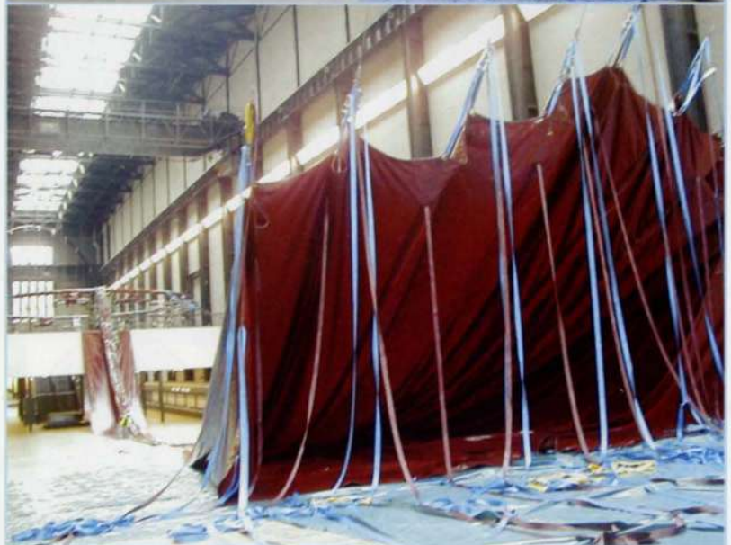
8. Raising membrane at east end.
