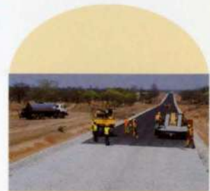
7. Surfacing unit with chip spreader about to lay the seal coat of 10mm stone.
