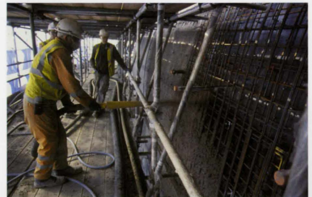
11. Spraying the substrate on site.
