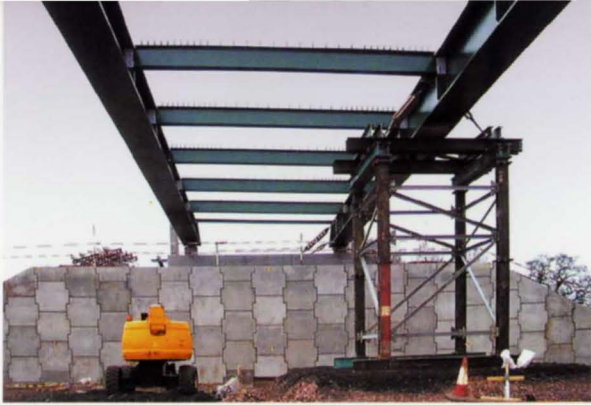
8. Simple, consistent design and construction: typical ladder beam deck and reinforced earth end-supports for two-span overbridges.
