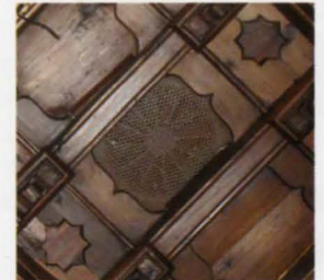
13. Ceiling panels with integrated air diffuser.
