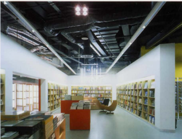
17. The bookshop, showing services integrated with structure.
