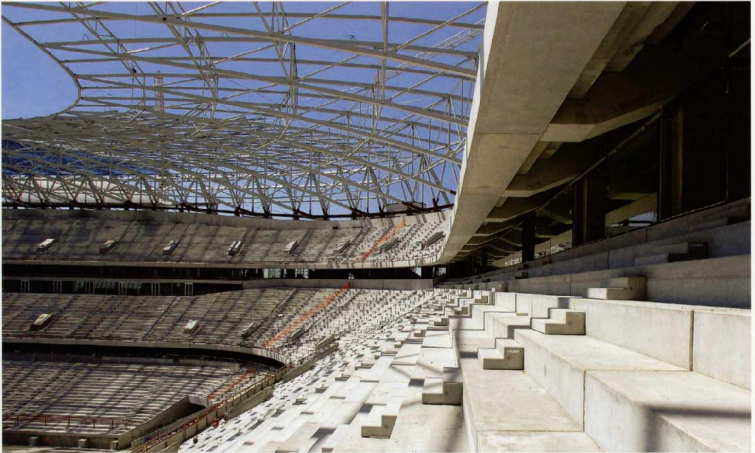
11. Bowl under construction, July 2004.
