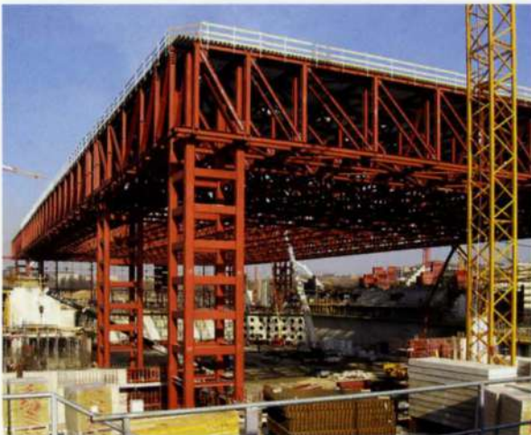
4. "Mega-columns" and roof under construction.
