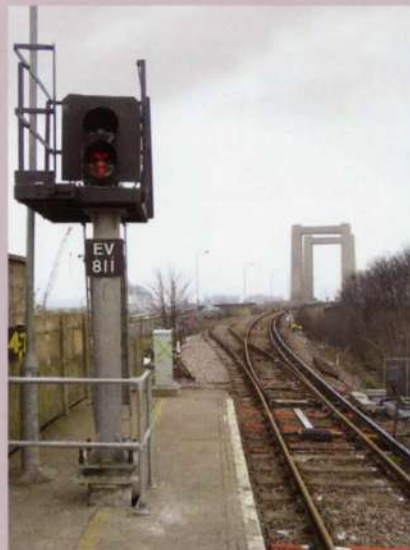
4. New two-aspect signal protecting the bridge just beyond Swale station.
