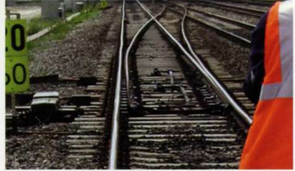
16. Ruscombe Junction on the GWR; the "kinks" in the track that contributed to its choice for analysis and study are clearly visible.
