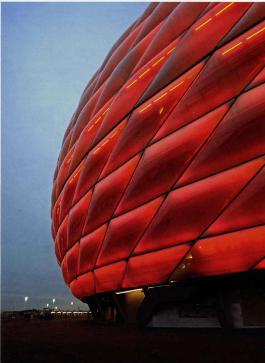
2. Stadium at dusk showing the ETFE pillows illuminated in the Bayern Munich colours.
