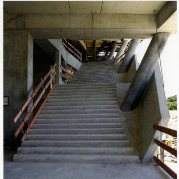
12. Cascading staircase under construction.
