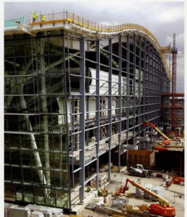
9. The south-west corner of the main terminal building.
