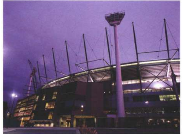
11. The Northern Stand structure at night.
