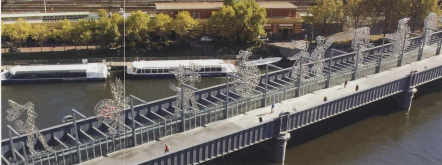
3. Sandridge Bridge from Freshwater Place on Southbank, showing the deck walkway for pedestrians and the adjacent former rail bridge section with its deck removed to expose the steel skeleton structure beneath. This view clearly reveals the bridge's marked skew across the river.
