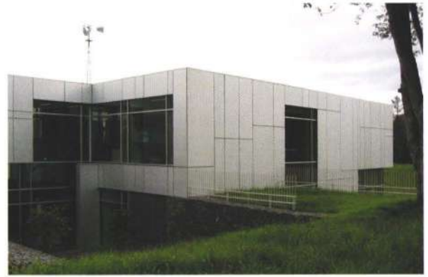
2. The new building is partially buried to further insulate against heat gains and losses.
