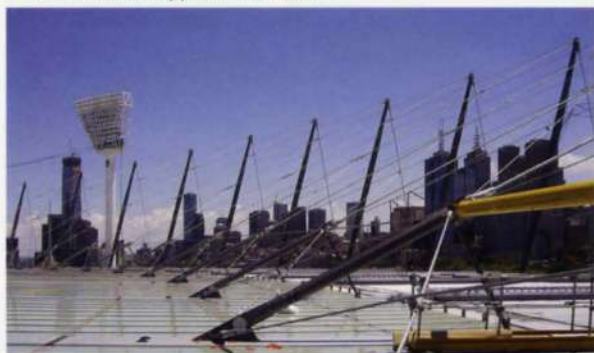
7. Cablenet supports to rafters.
