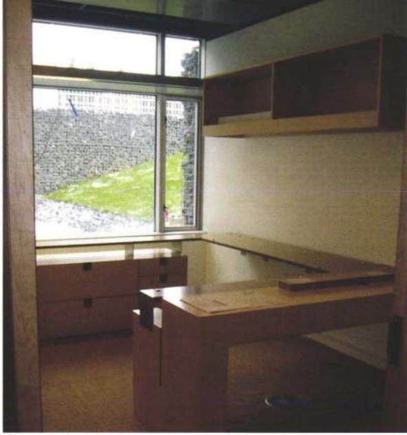
7. Airflow from the floor diffusers in the offices is integrated within the furniture locations and can be manually adjusted.
